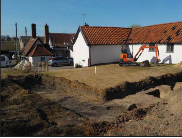
1 View of site looking north
