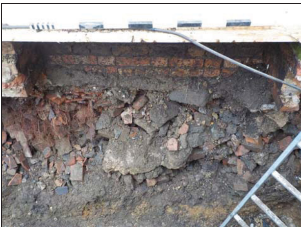
5 Sample Section 3 looking south
