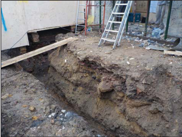
1 General view of trench looking west
