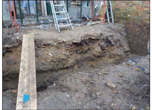
2 General view of trench looking north-west
