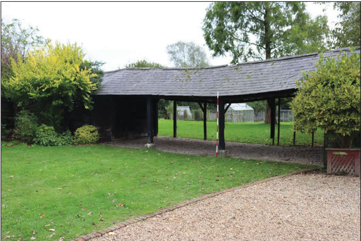
Plate 2 North-west elevation showing open-fronted section (Unit 2), taken from the west (DP03)
