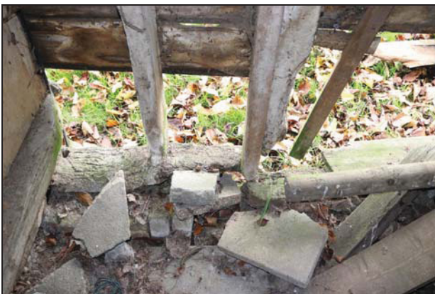
South-east wall of Unit 3 showing primary-braced framing, taken from the north-west
