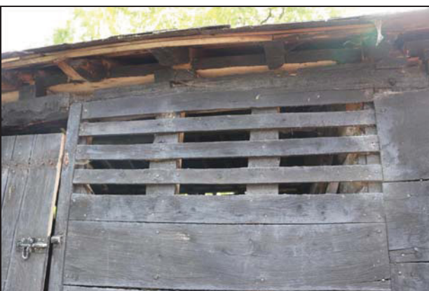
DP 15 North-west elevation (Units 3 and 4) showing wide horizontal boarding with ventilation apertures, taken from the south-west
