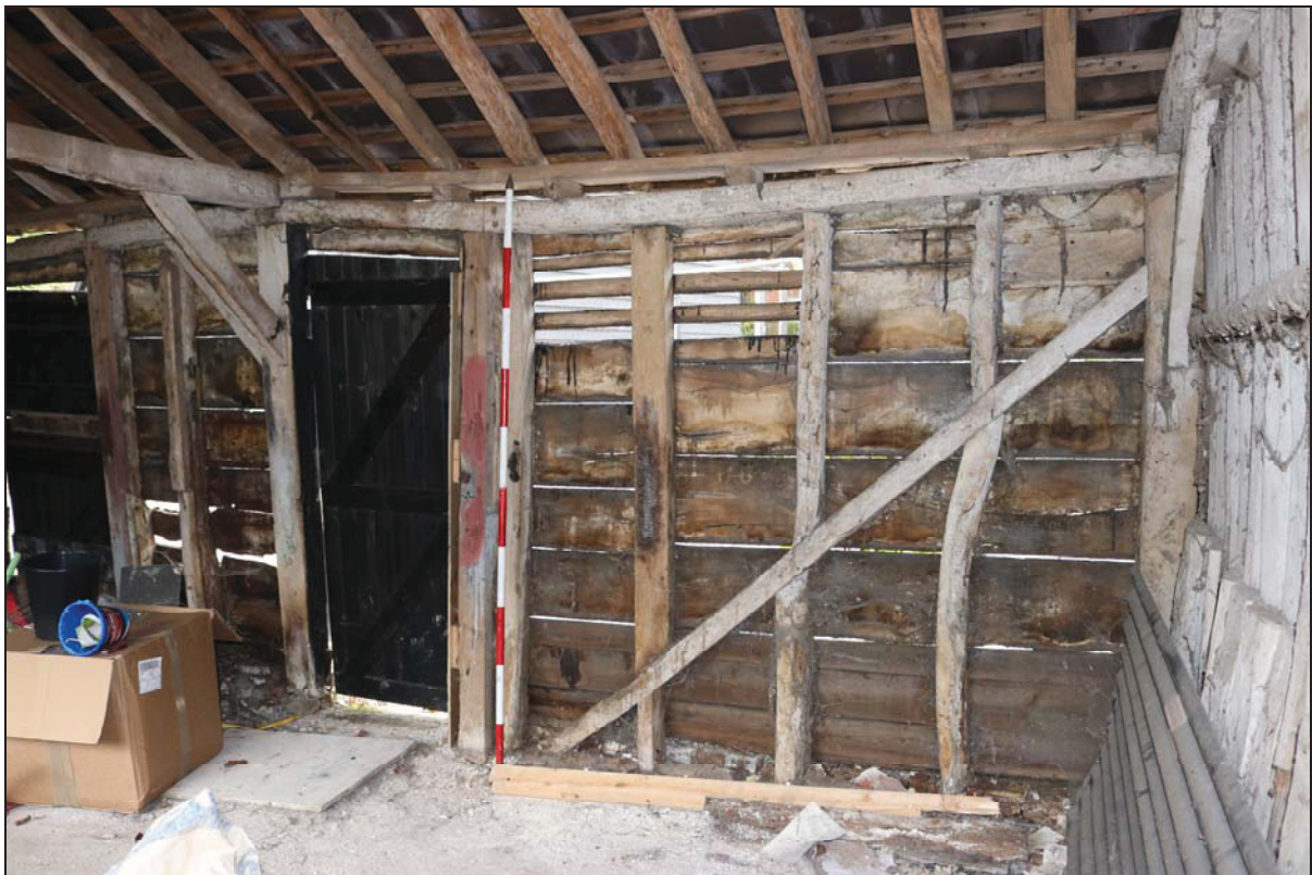
Plate 8 North-west wall of Unit 5 (north-east bay), taken from the south-east (DP 81)
