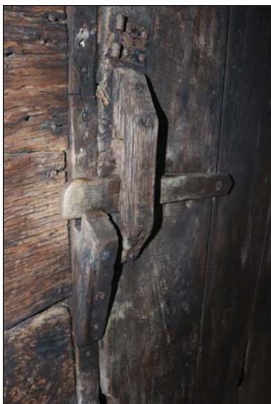
Detail of the boarded door (Unit 1) with early timber latch, taken from the west
