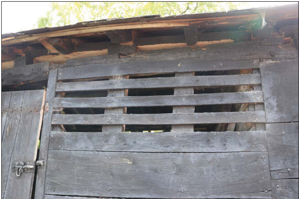
Plate 4 North-west elevation (Unit 3) showing ventilation aperture, taken from the north-west (DP 17)
