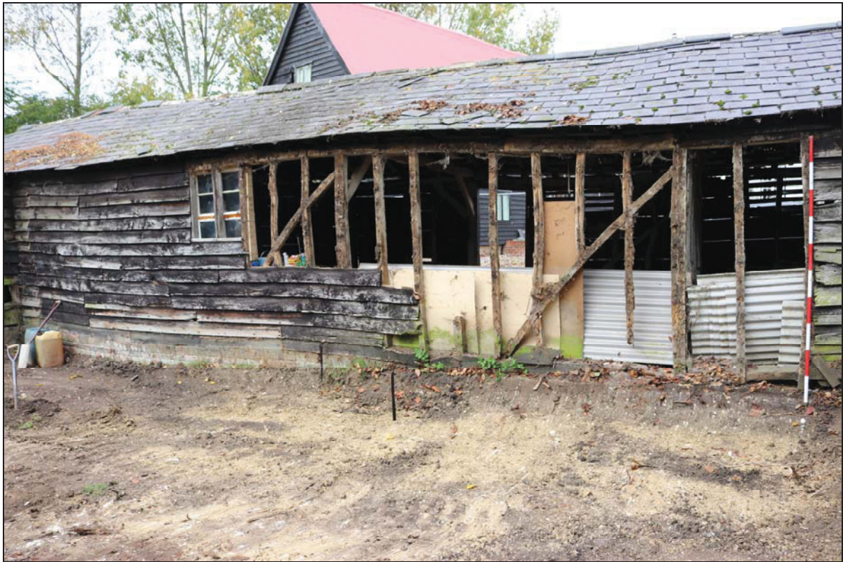
Plate 5 South-east elevation (Unit 5), taken from the south-east (DP 12)
