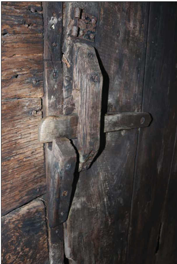
Plate 10 Detail of the boarded door (Unit 1) with early timber latch, taken from the west (DP 41)
