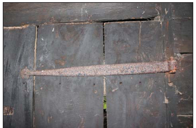
Outer face of the historic boarded door (Unit 1) with early hinges and timber latch, taken from the south-west
