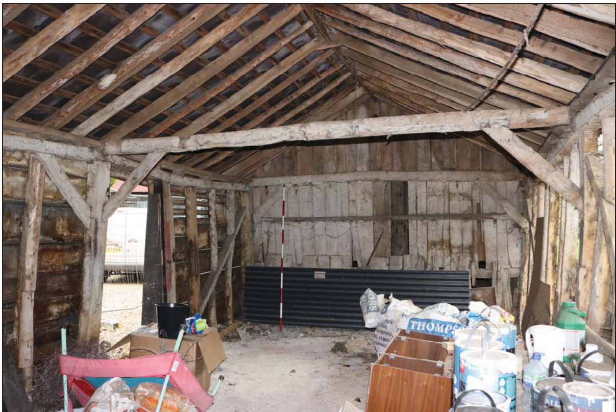
Plate 18 Interior of Unit 5, taken from the south-west (DP 78)
