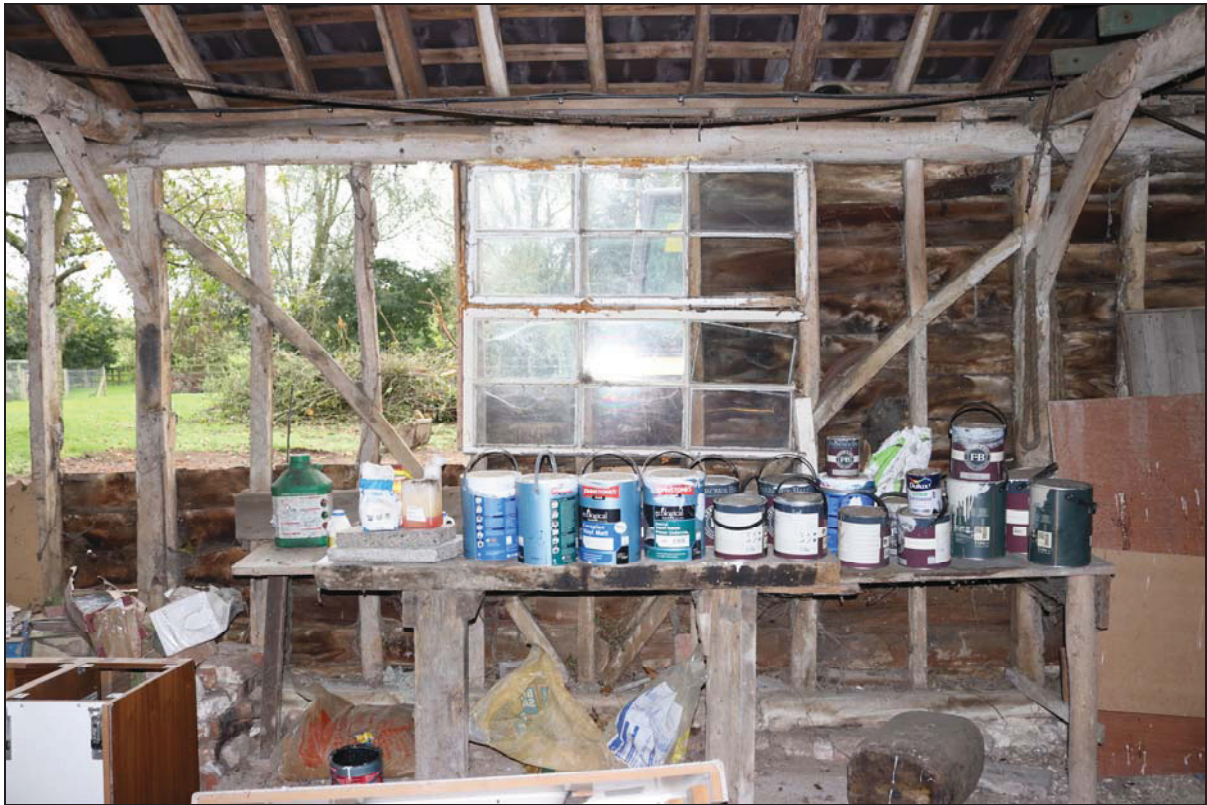
Plate 7 South-east wall of Unit 5 (central bay), taken from the north-west (DP 91)
