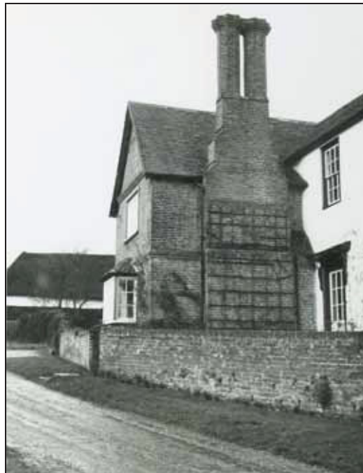
4.2 View of the 17 th century brick addition to the main farmhouse. Source: Website 1
