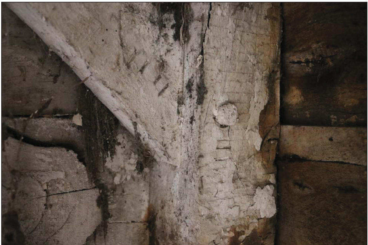
Plate 16 North-east corner of Unit 4 showing pegged inner brace with assembly marks, taken from the south (DP 77)
