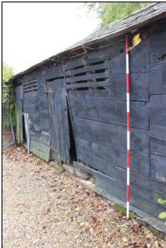
DP 15 North-west elevation (Units 3 and 4) showing wide horizontal boarding with ventilation apertures, taken from the south-west
