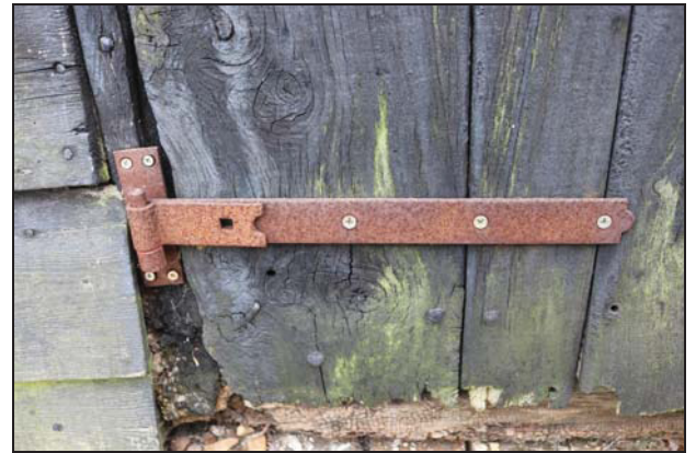
DP 20 Detail of the door on the north-west elevation (Unit 4) showing original pintle and impression of strap hinge, taken from the north-west
