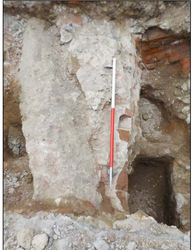
12 Wall 1016 in plan view showing concrete encased pipe cutting through on the left
