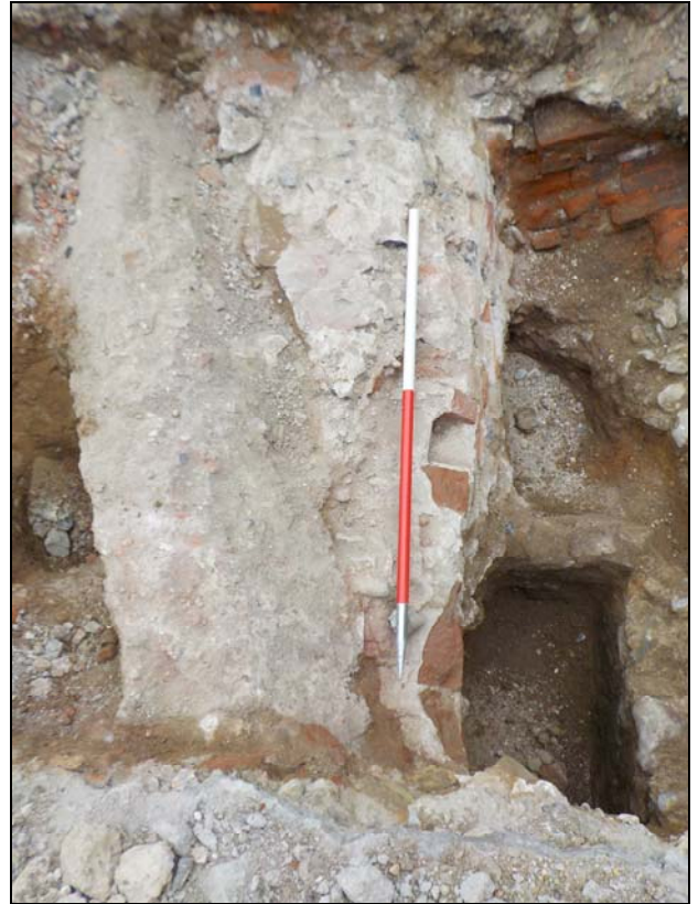
12 Wall 1016 in plan view showing concrete encased pipe cutting through on the left
