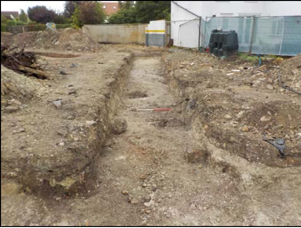
11 View of Trench 3 looking west
