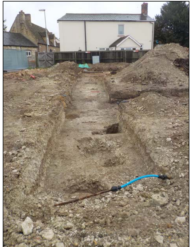
10 View of Trench 3 looking south
