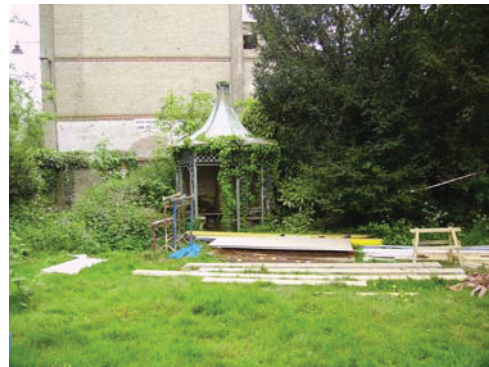
DP4 Listed gazebo in Mill House garden. From N
