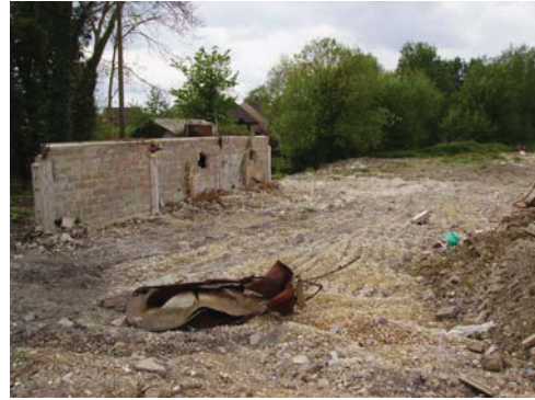
DP2 Sub-station wall, with river channel behind. From NE
