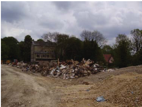
DP3 Parkers Mill on eastern site boundary, partially obscured by mounds of waste. From NW
