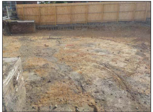
10 General view of Trench 3 looking north-east
