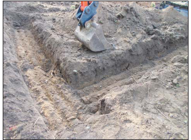
4 South-east corner of footings
