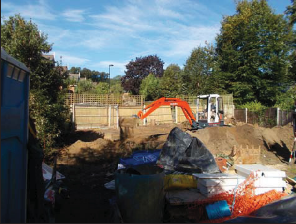
1 Site being excavated
