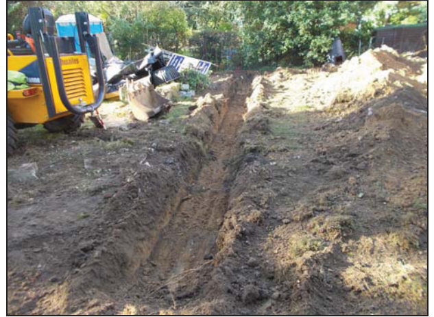
2 Southern edge of footings
