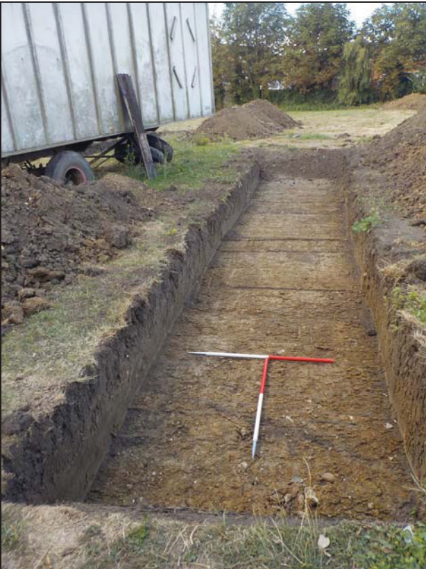
19 Trench 4A looking south-west
