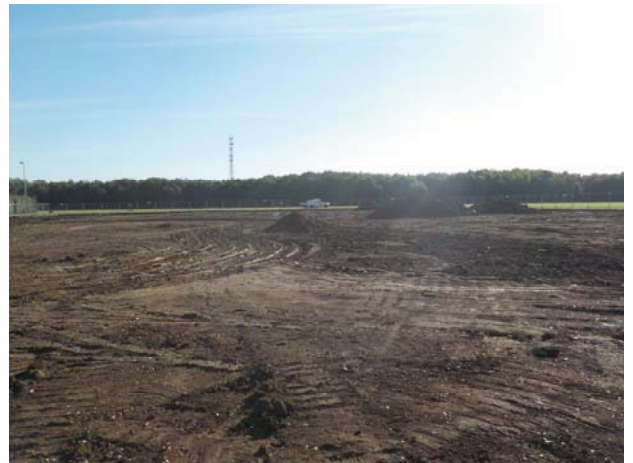
4 Site after removal of topsoil
