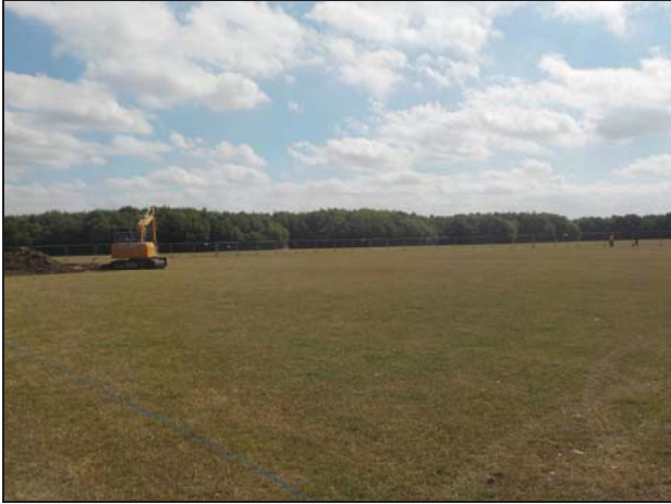
1 General view of site before commencement of topsoil strip
