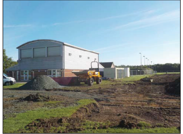
2 General site view during removal of topsoil
