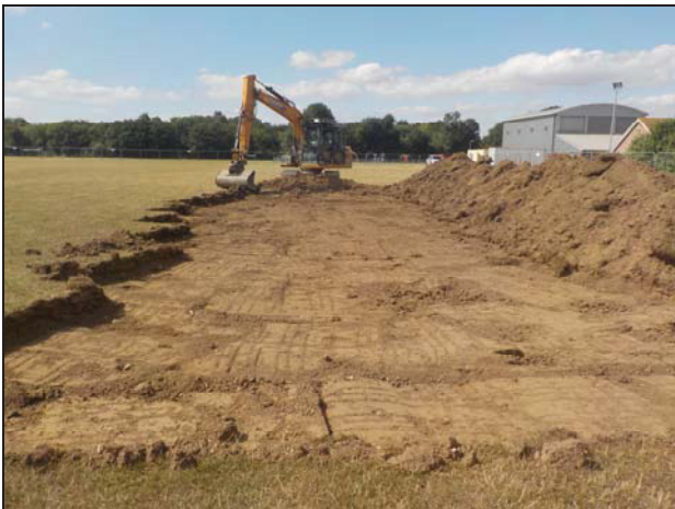
3 Removal of topsoil
