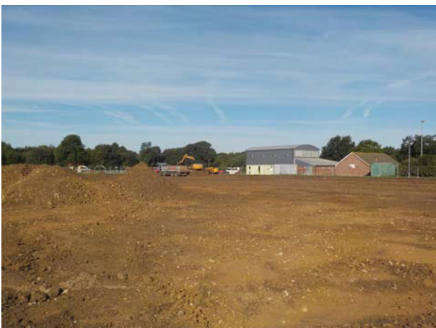
5 Site after removal of subsoil
