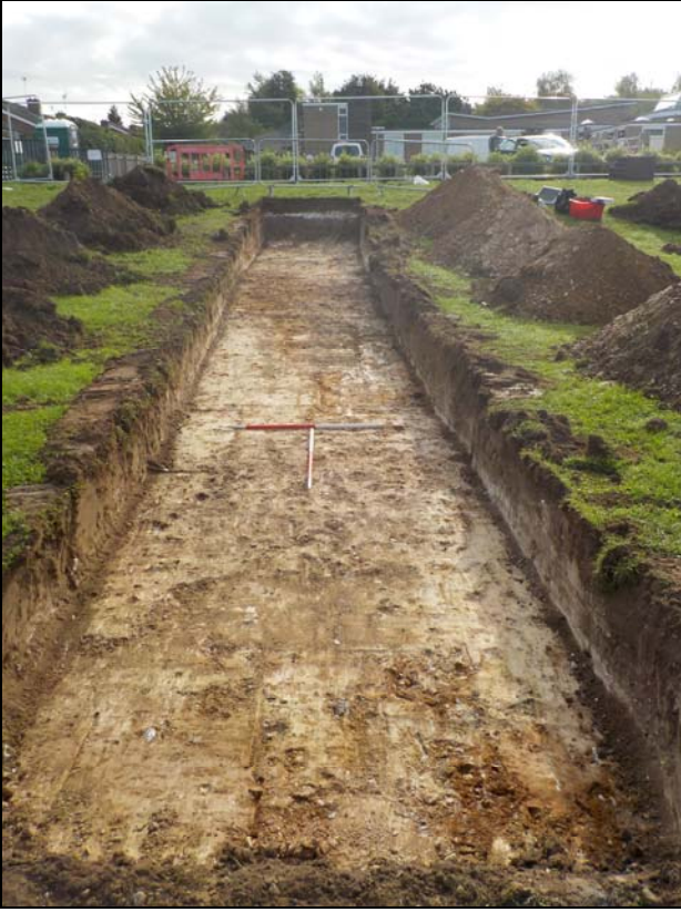
1 Trench 1 looking east
