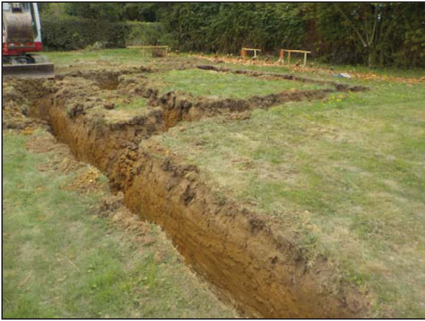
5 Area 1 looking north-west
