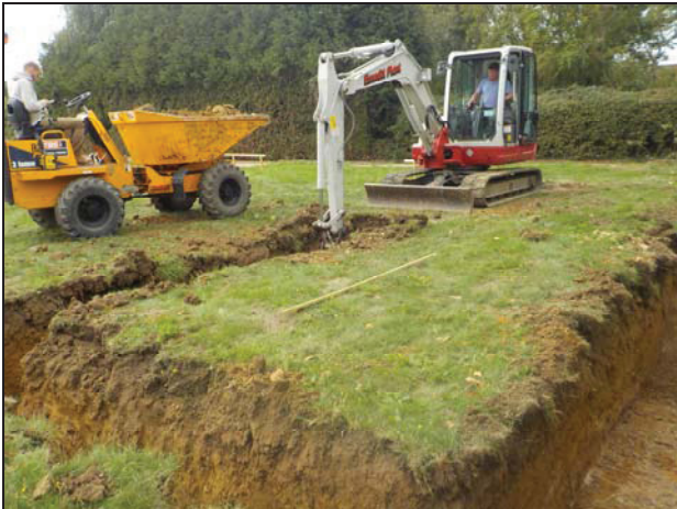
3 Excavation of footings looking south-west
