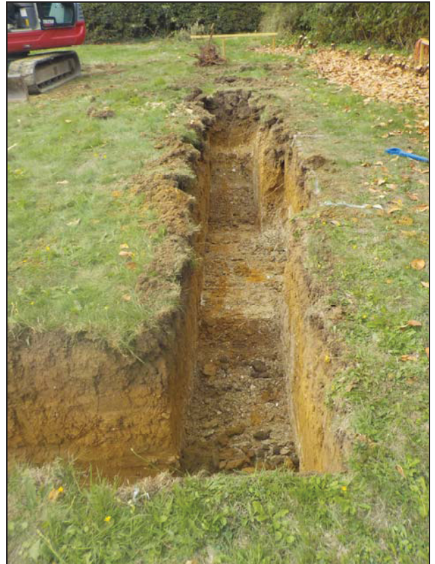
4 Excavated footings looking west
