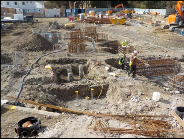
46 Excavation of Monitoring Test Pits March 2018
