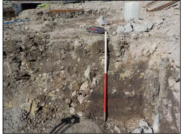
47 Monitoring Test Pit 1
