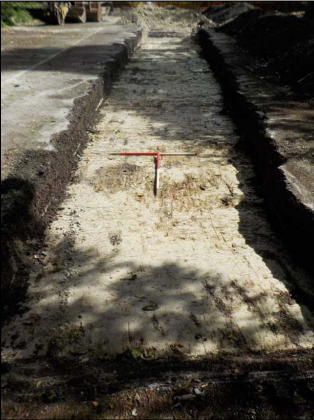
13 View of Trench 8 looking north-east
