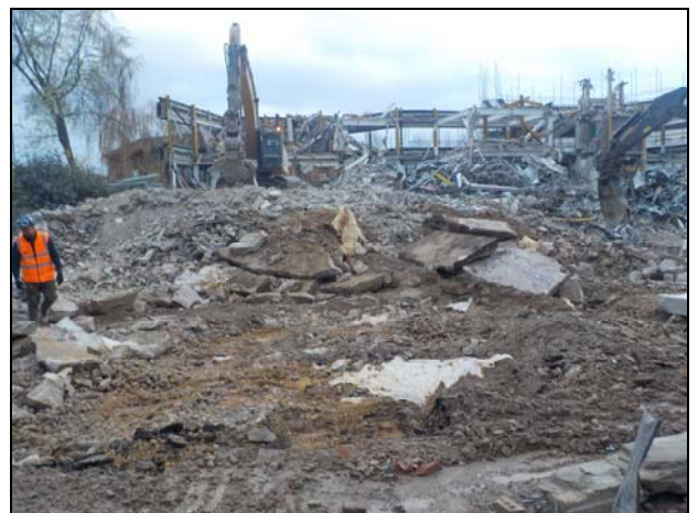
45 Monitoring of demolition work November 2017
