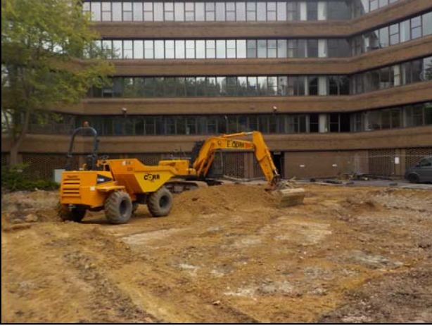
22 Excavation area being stripped
