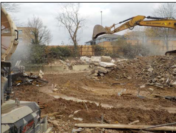
44 Monitoring of demolition work November 2017
