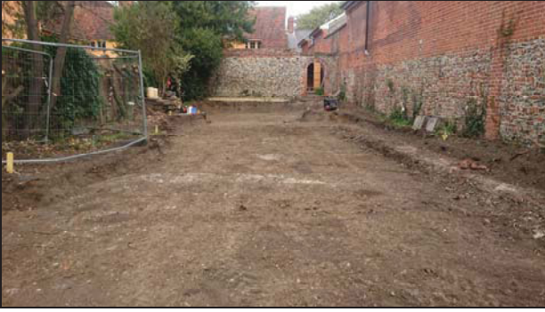
1 General site overview looking north-west
