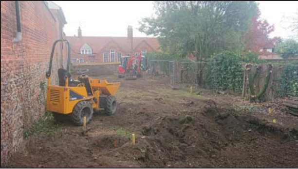
3 Initial ground reduction looking south
