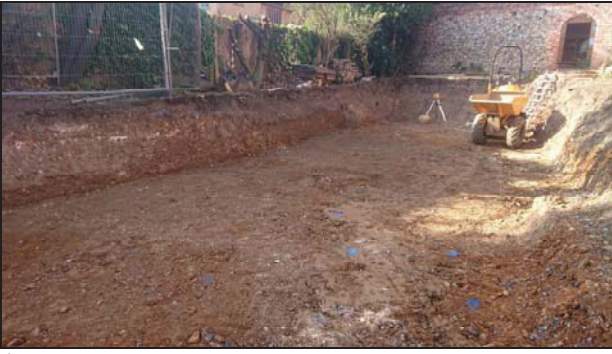
17 Completed ground reduction looking west
