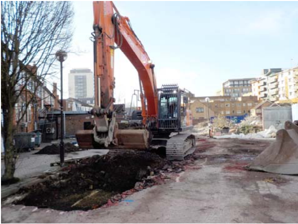
7 Trench 4 being machined showing services
