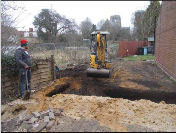
Excavation of footing trench looking east.
