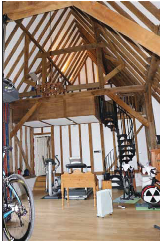
Plate 12 Truss 2 in Barn 1, taken from the south (DP 27)
