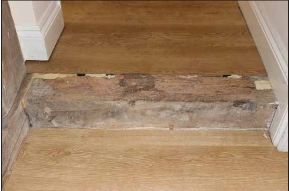
Plate 13 Surviving sole-plate of the original north-east end wall of Barn 1, taken from the south-west (DP 60)
