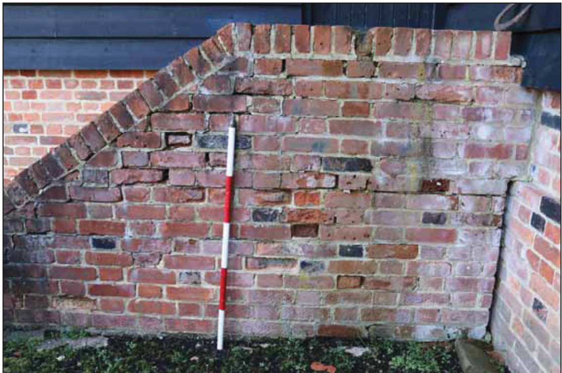
Plate 4 Steps giving access to the north-west extension of Barn 1, taken from the south-west (DP 11)
