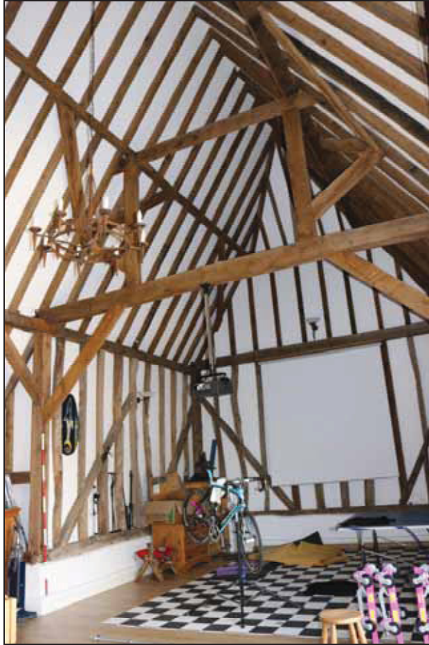
Plate 5 Truss 1 in Barn 1, taken from the north (DP 26)
