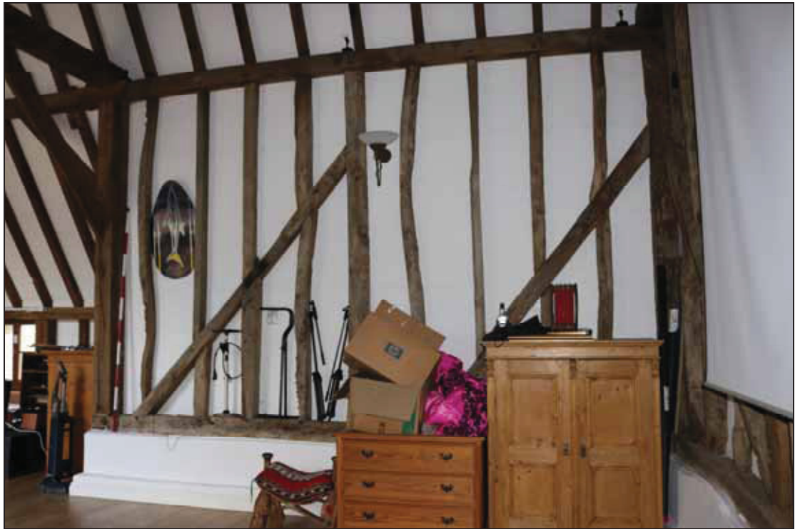
Plate 7 South-east side of bay 1 in Barn 1, taken from the west (DP 41)
