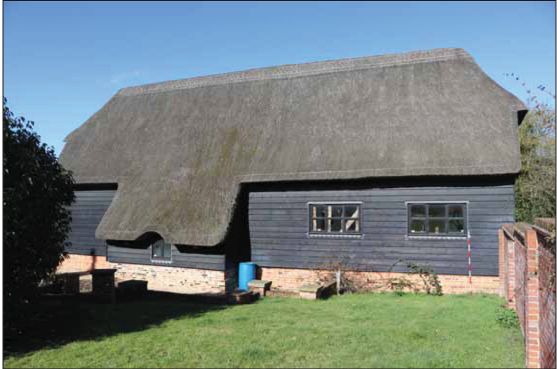
Plate 3 South-east elevation of Barn 1, taken from the east (DP 01)
