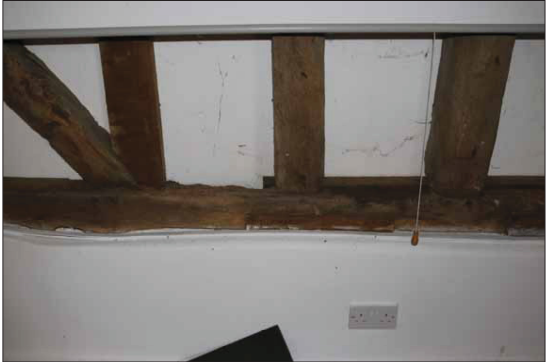
Plate 9 Studwork and sole-plate at the south-west end of Barn 1, taken from the north-east (DP 40)
