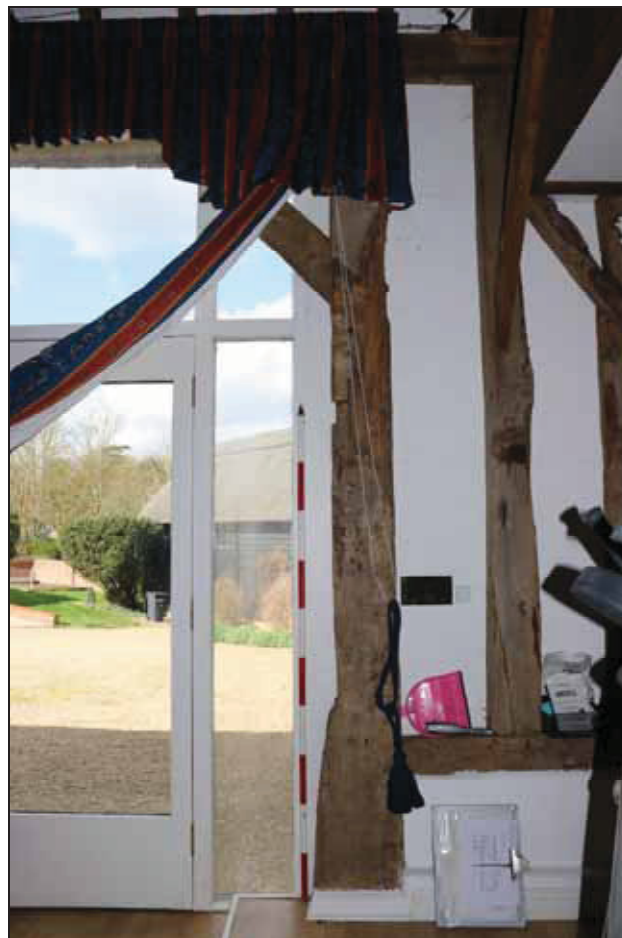
Plate 10 North-west side of bay 2 in Barn 1, taken from the south-east (DP 31)
