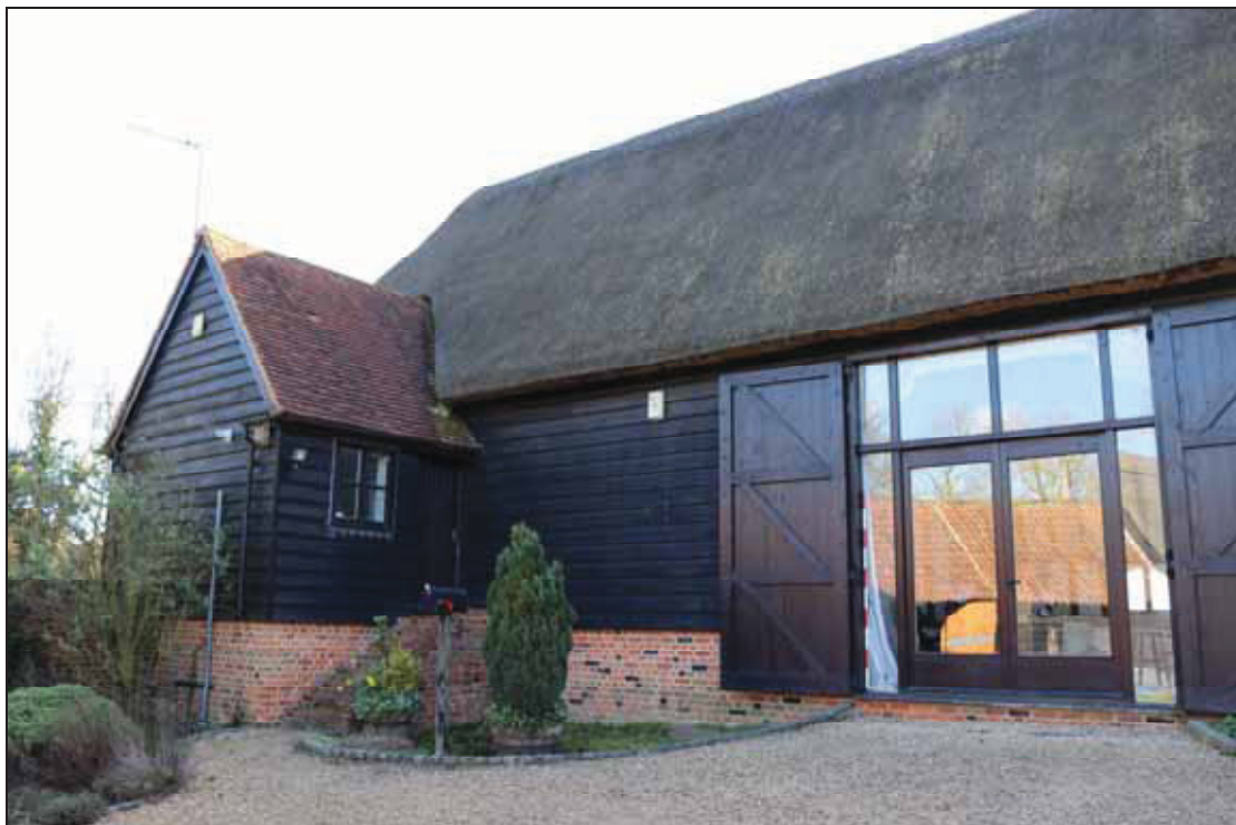
Plate 2 Exterior of Barn 1, taken from the west (DP 03)
