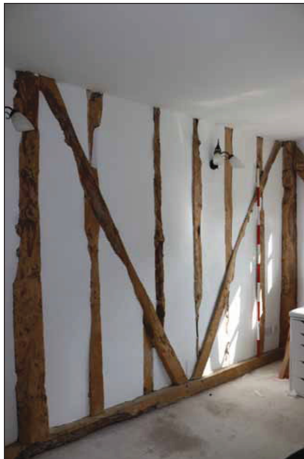
Plate 14 North-east end of bay 3 in Barn 1, taken from the south-west (DP 48)
