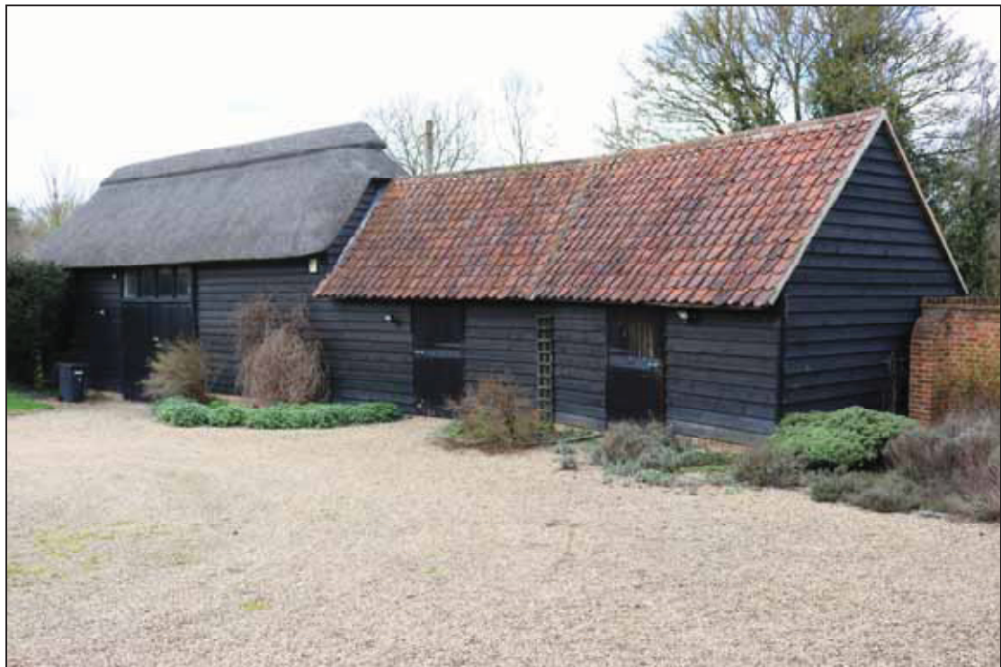
Plate 16 Exterior of Barn 2, taken from the south-east (DP 07)
