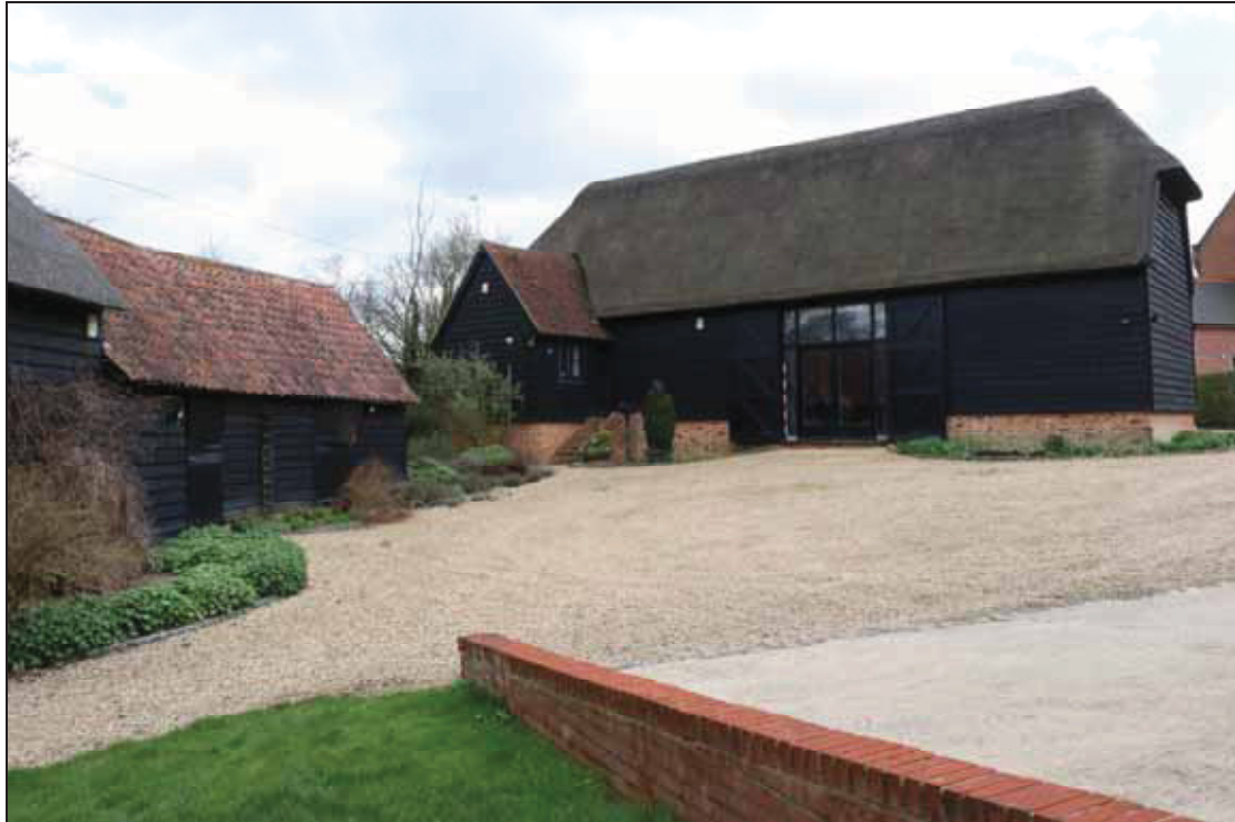
Plate 1 Exterior of the barns, taken from the west (DP 05)
