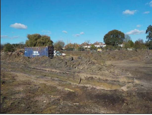
1 General view of site looking north
