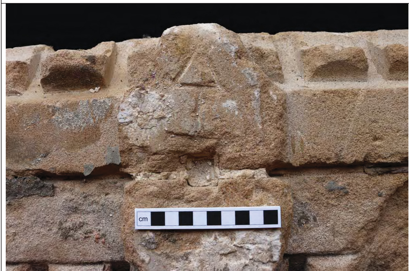
Detail: top of mullion showing mason's mark
