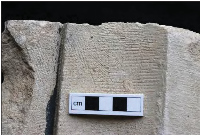
Detail of tooling marks
