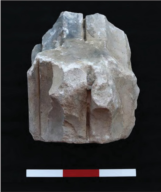
Side with glazing groove
