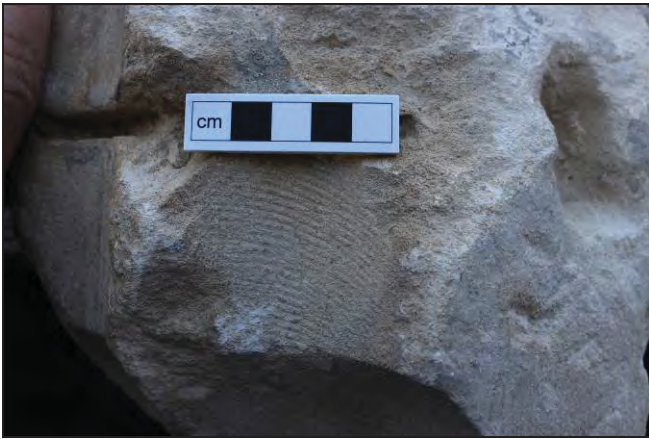
Detail of fine tooling
