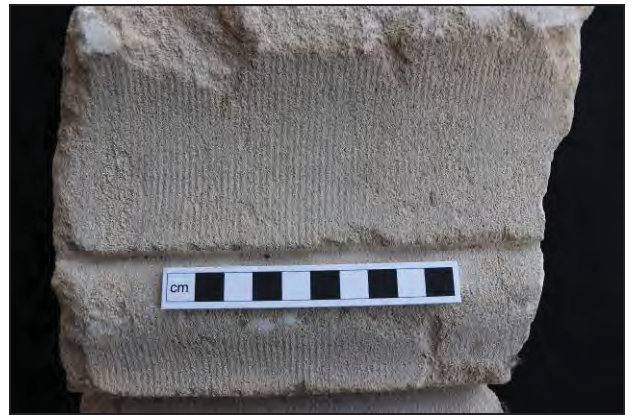
Detail: tooling marks
