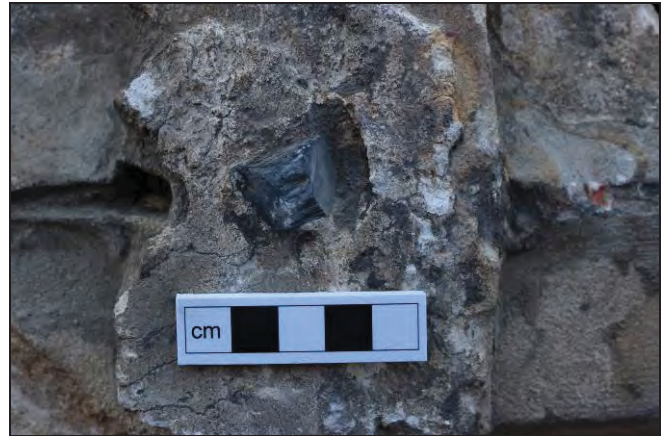
Detail of top with lead filled socket
