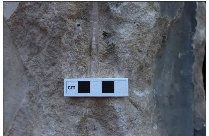
Detail of glazing groove
