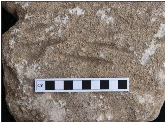
Detail showing tooling marks
