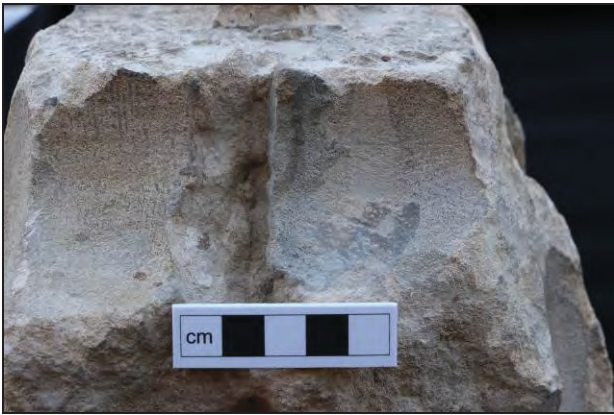
Detail of glazing groove
