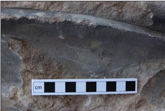
Detail of tooling marks
