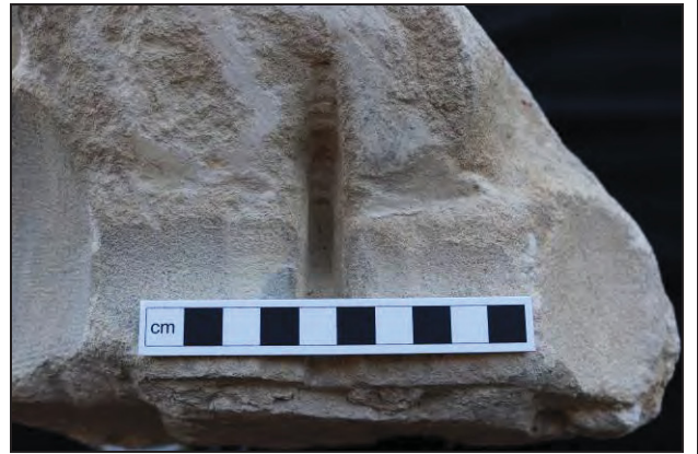
Detail of glazing groove
