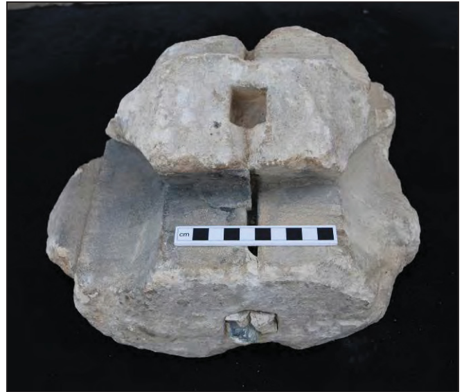
Oblique view with sockets and glazing grooves
