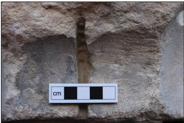
Detail of glazing groove
