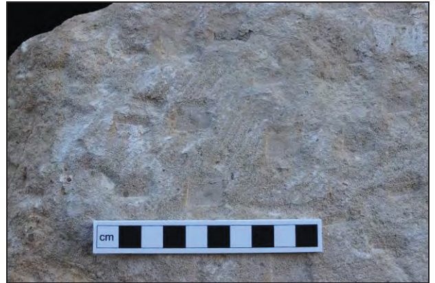
Detail of the tooling marks
