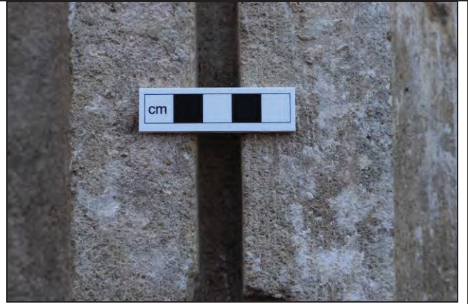
Detail of the wide glazing groove
