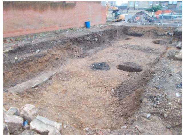
DP 4. South part of Area A. Looking south-west.
