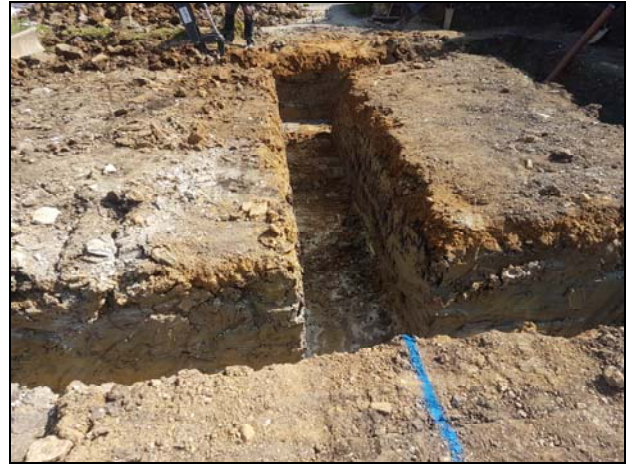
4 Site during excavation of footings looking east
