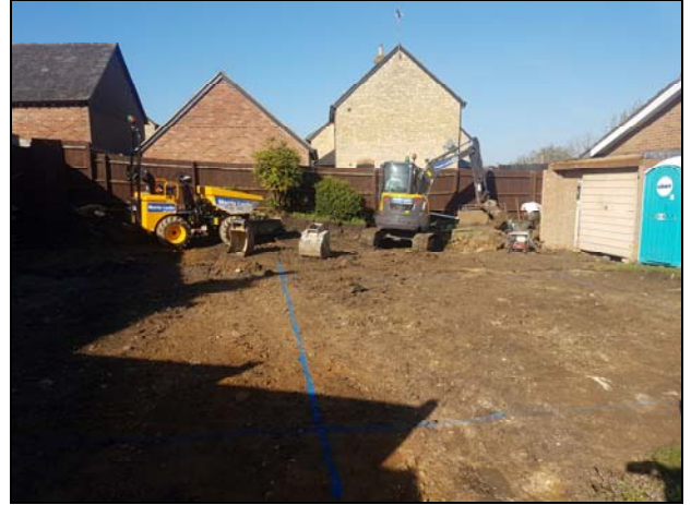
2 Site prior to excavation of footings looking west
