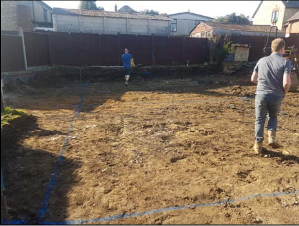
1 Site prior to excavation of footings looking south
