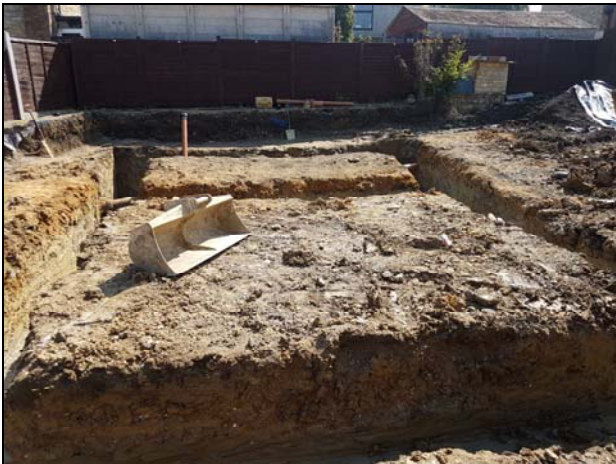
13 Site following excavation of footings looking south
