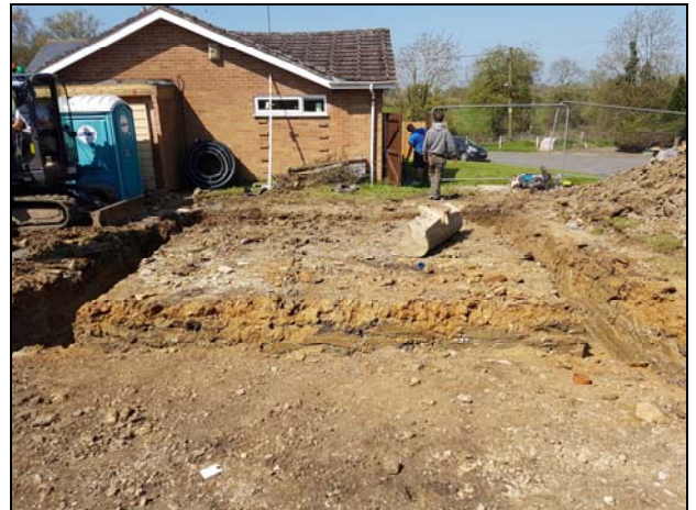
14 Site following excavation of footings looking north
