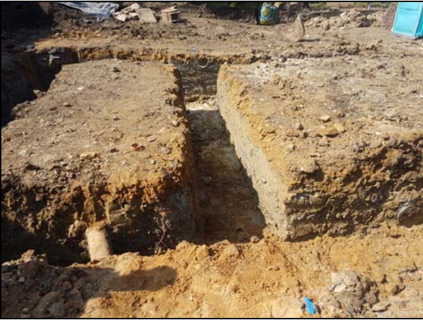
3 Site during excavation of footings looking west
