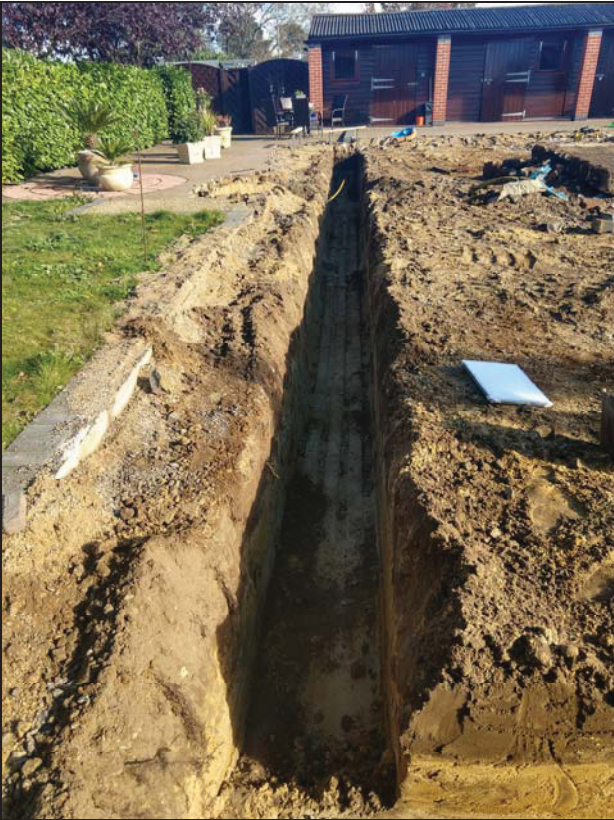
3 North-western footing looking east
