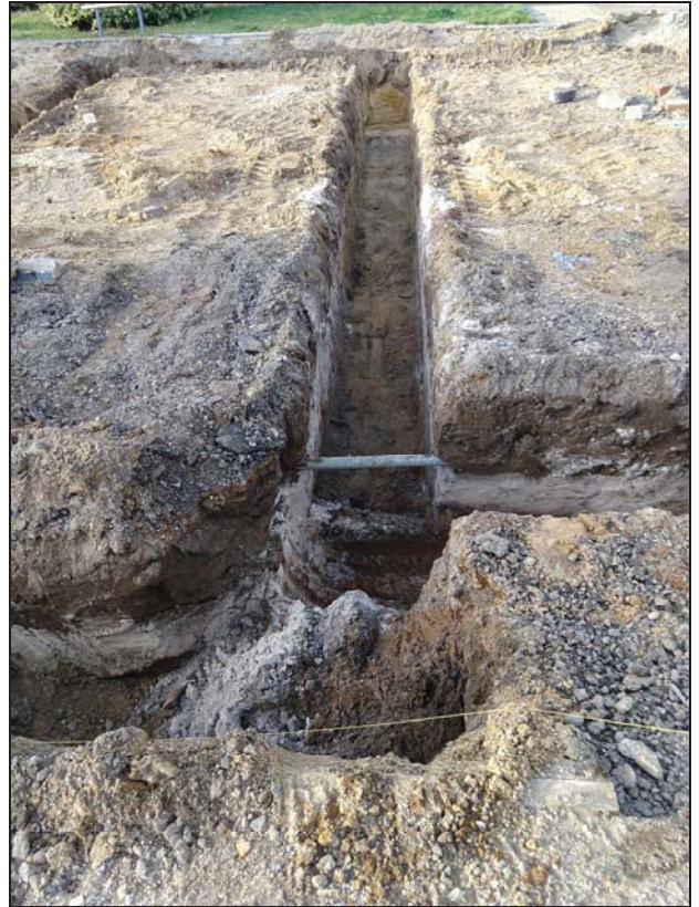
4 Services seen in central footing cut looking north
