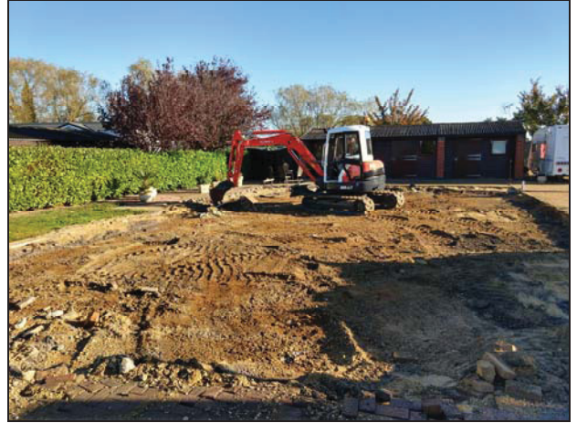
2 General site overview looking east
