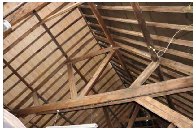
DP 56 East wall-plate of Bay 4 (barn) showing scribed Baltic timber mark obscured by electrical wiring (indicated), taken from the west
