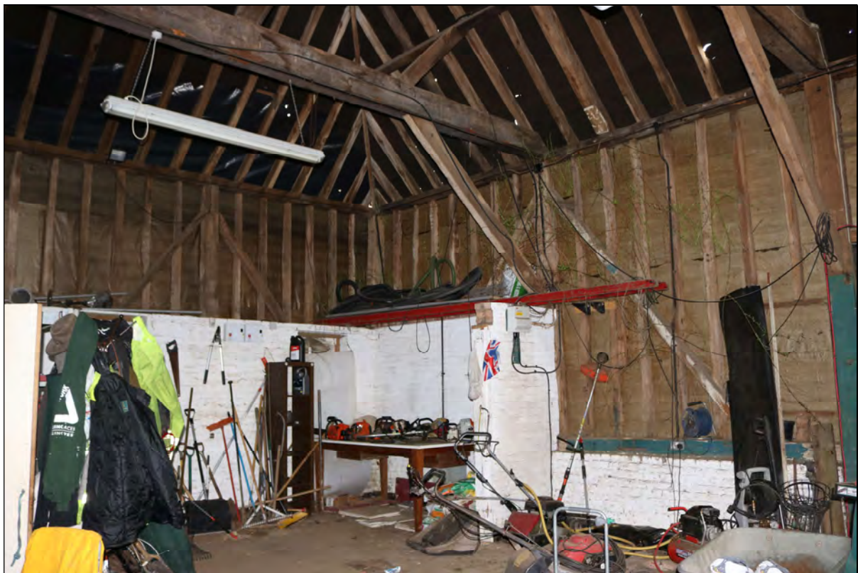
Plate 8 North-east former of the barn, taken from the south-west (DP 7)
