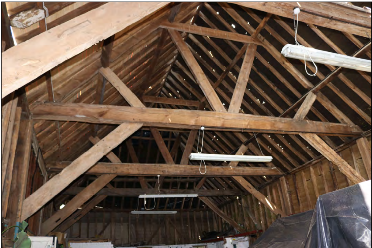
Plate 6 Roof structure over the barn, taken from the south (DP 40)
