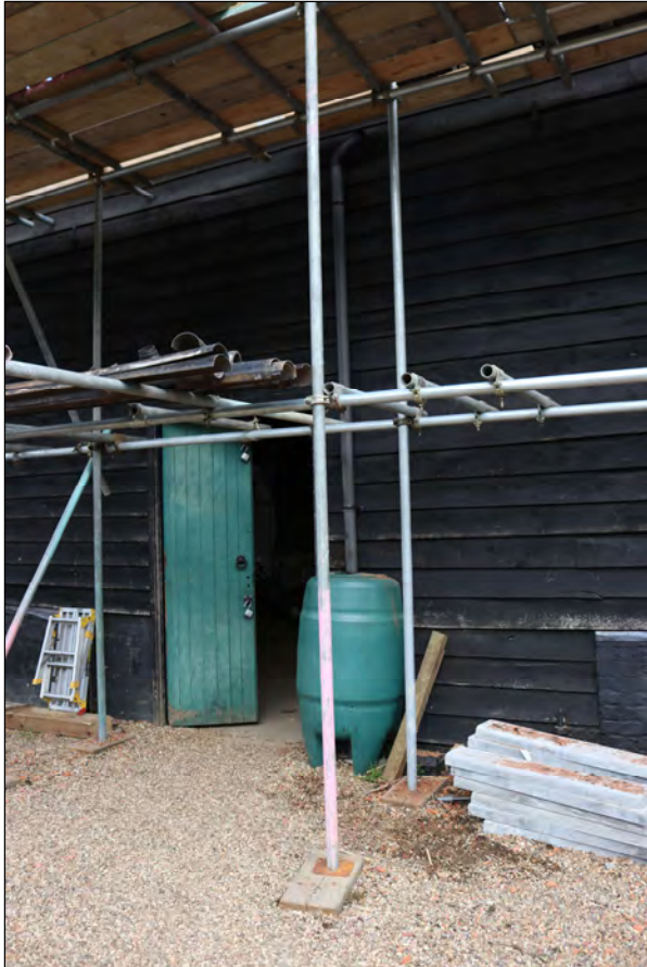
Plate 3 Entrance on the west side (barn) showing doorway set in former larger threshing doorway, taken from the south-west (DP 6)
