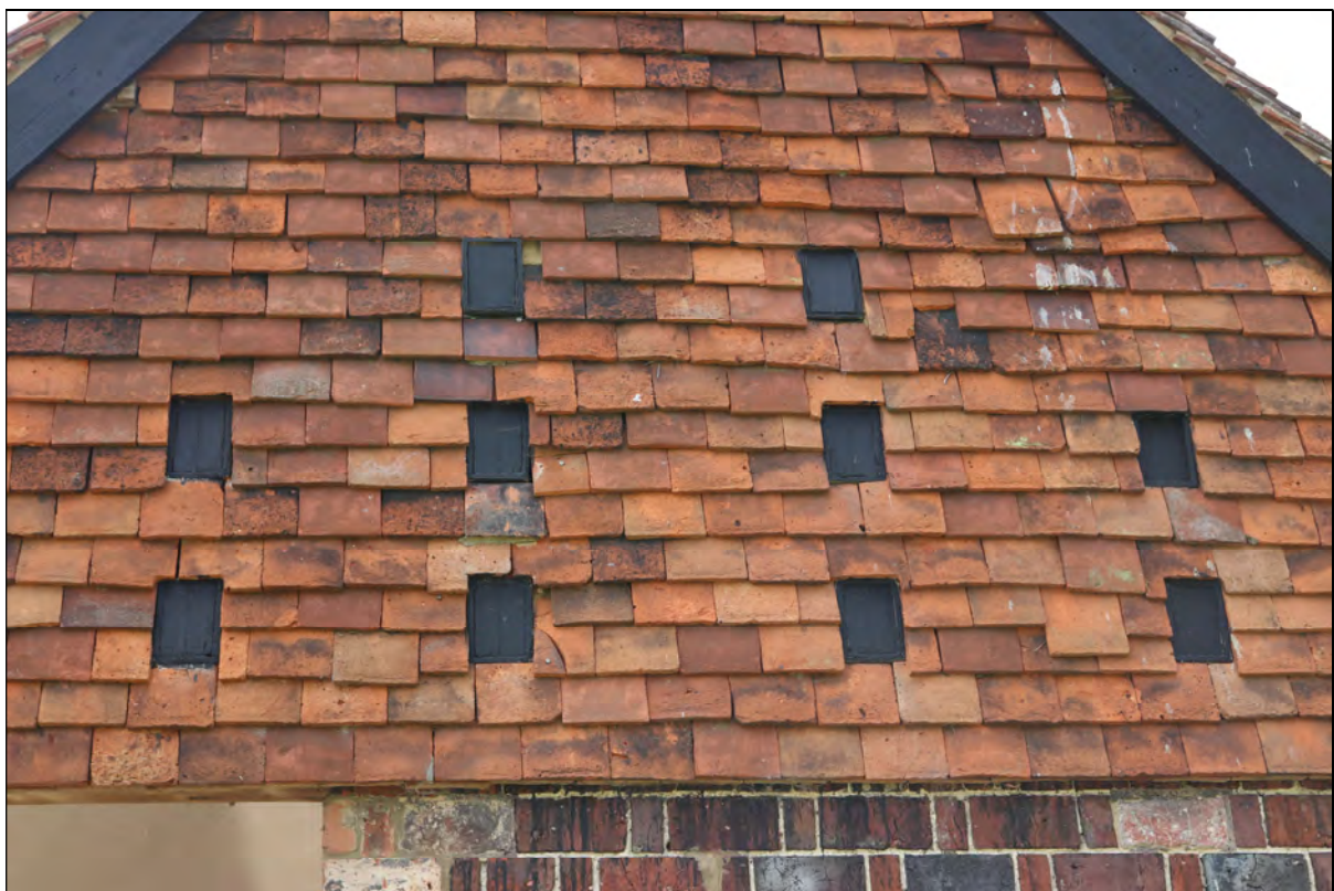
Plate 16 East elevation (cart-shed) showing small blocked apertures likely marking a dove-cote, taken from the east (DP 13)
