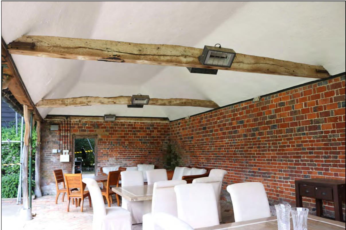
Plate 17 Interior of the cart-shed, taken from the east (DP 20)
