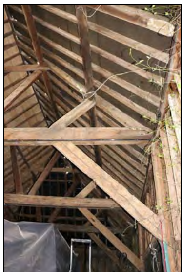
DP 59 East end of Truss 3 (barn), taken from the south
