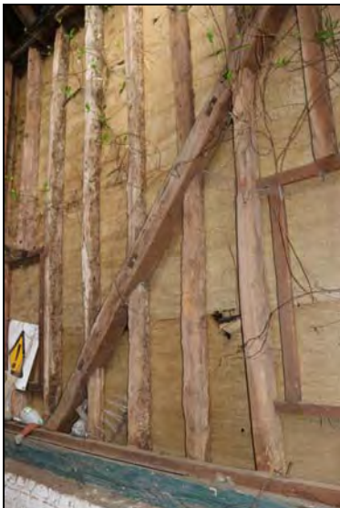
DP 57 East wall of Bay 4 (barn) showing reused timber as a primary-brace, taken from the south-west
