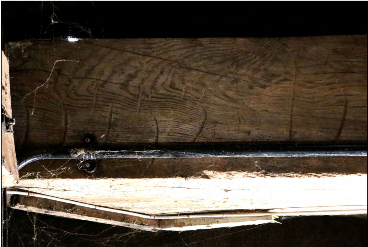
Plate 11 Soffit of the tie-beam (barn: Truss 2) showing scribed Baltic timber mark "33453 | 3" (DP 50)
