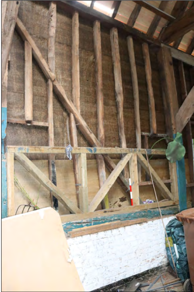
Plate 7 West wall of Bay 4 (barn) showing primary-braced framing, taken from the south-east (DP 69)
