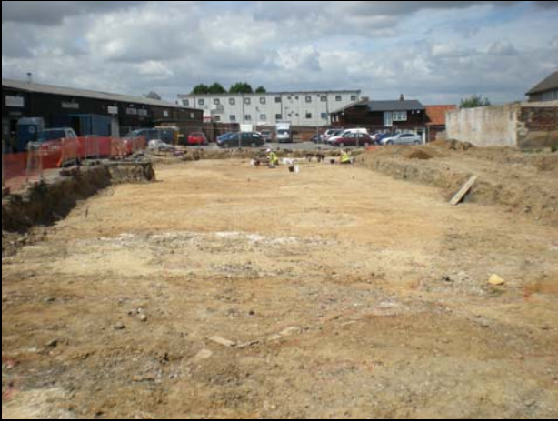
1 Overview of excavation area
