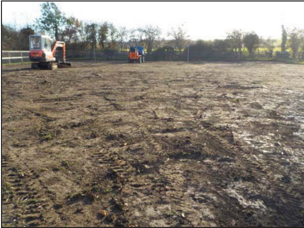
3 Area of excavation looking east
