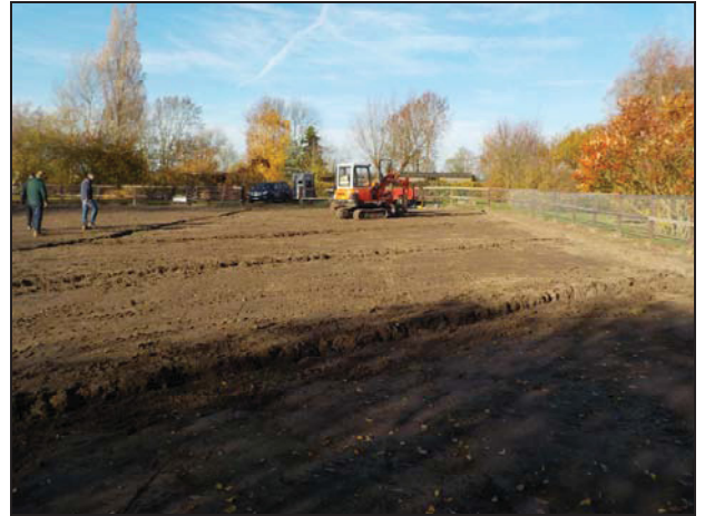
4 View of excavated drainage channels looking north
