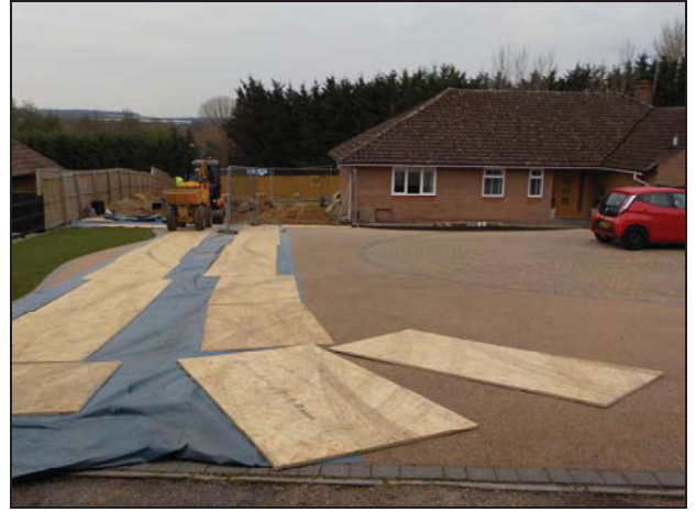
2 General site overview looking south-east
