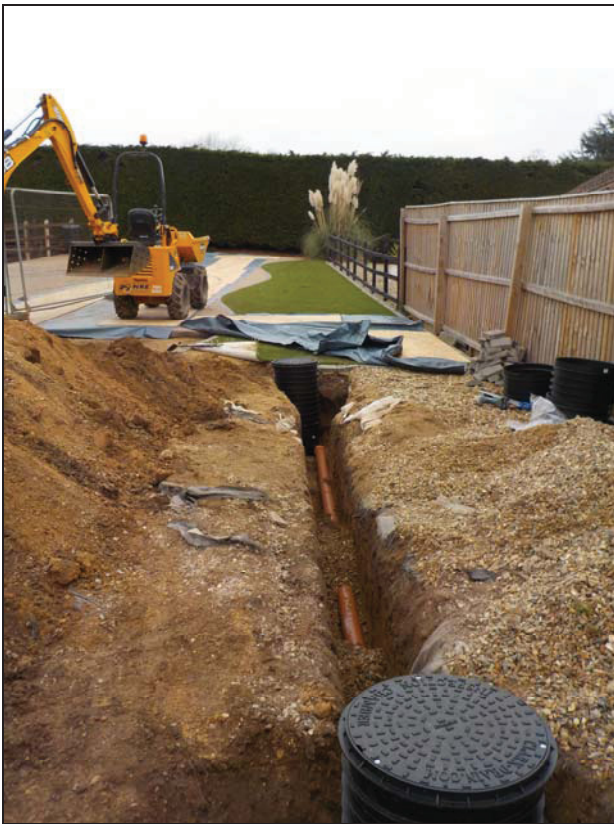
3 Cut of service trench looking north-west
