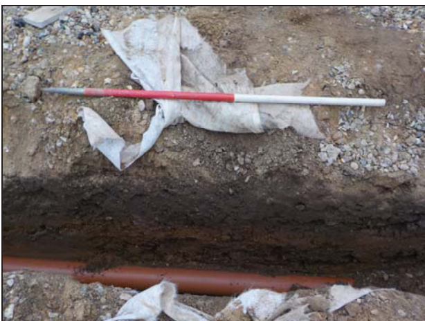
5 Sample Section 2 looking east
