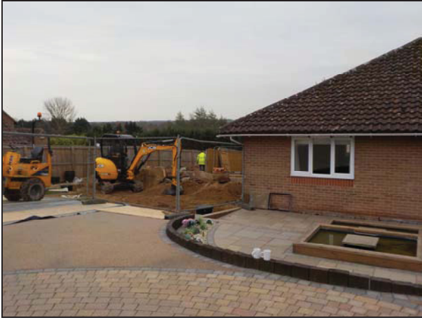
1 General site overview looking south
