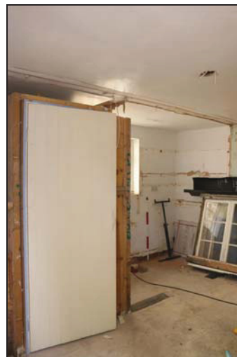
DP 6 Utility room during the planned works, taken from the north
