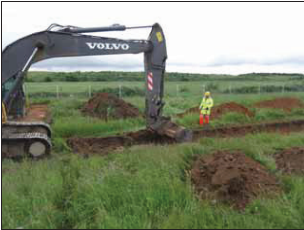
1 Cutting of trenches, facing southwest
