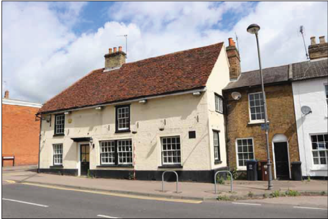
Plate 1 Exterior of Building 1 and Building 2, taken from the south-east (DP 01)
