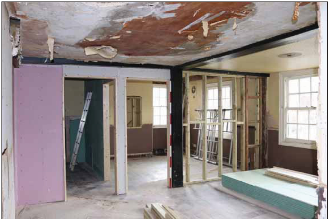
Plate 6 Interior of GF01 in Building 1, taken from the north-west (DP 34)
