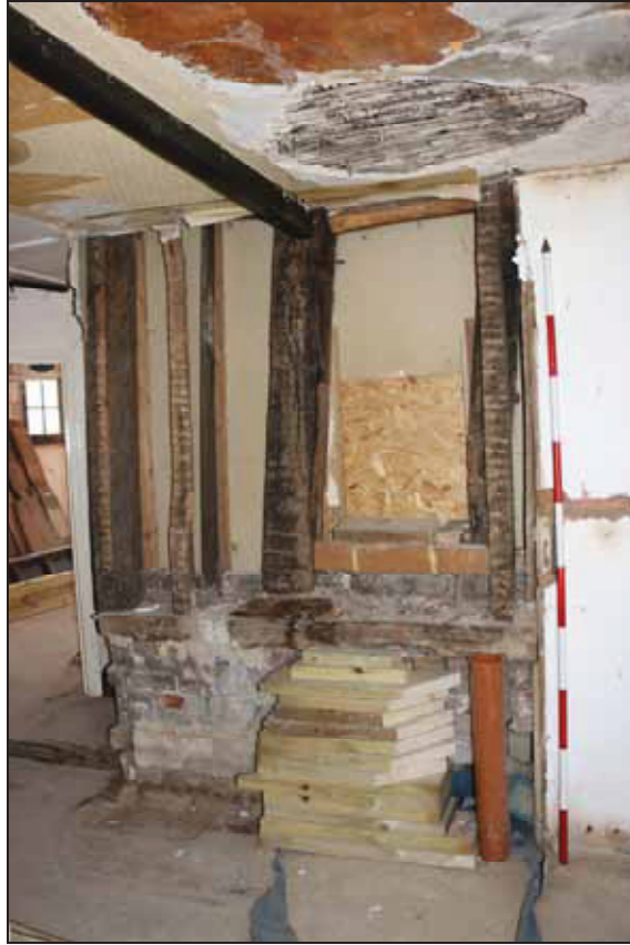
Plate 7 Timber-framing in GF01 in Building 1, taken from the south (DP 31)
