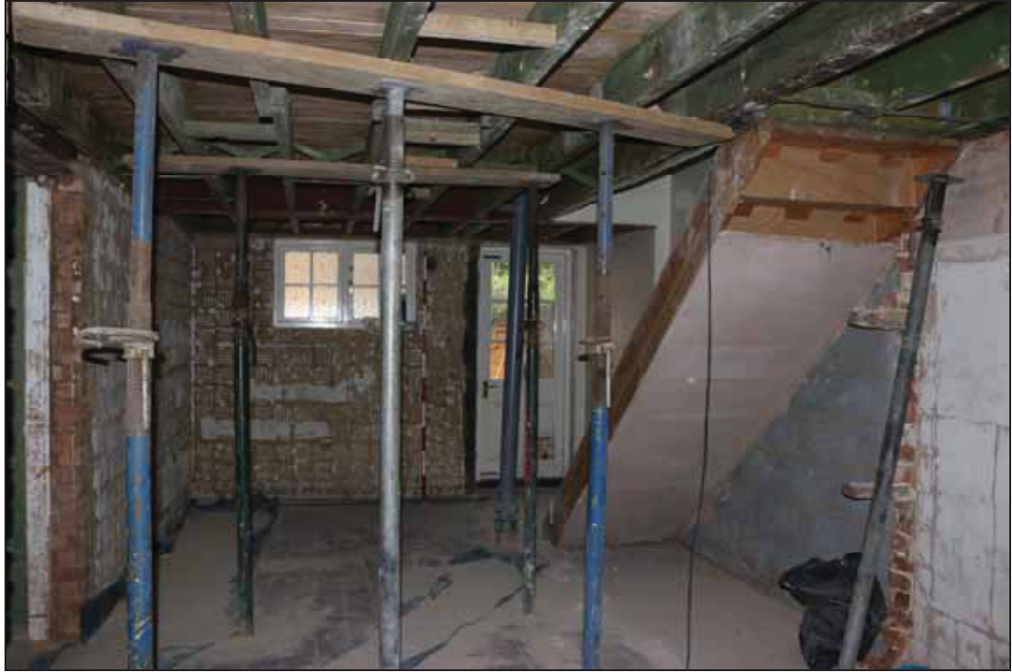
Plate 27 Interior of Building 2, taken from the south (DP 49)
