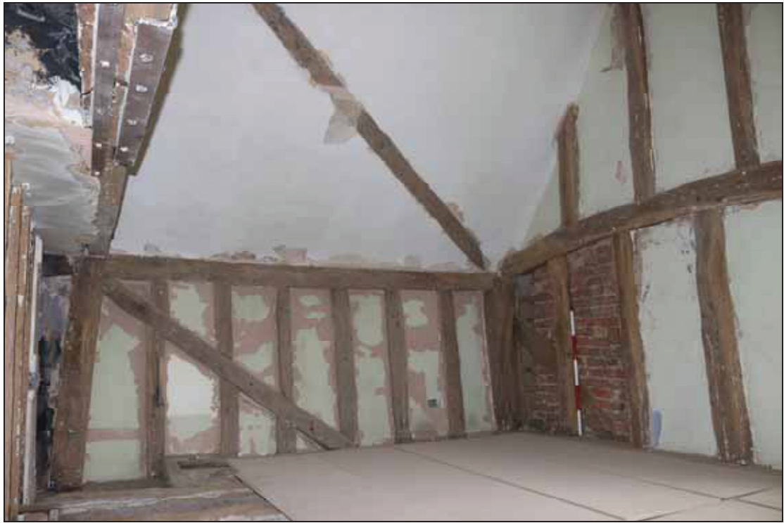
Plate 21 Timber-framing in FF04 in Building 1, taken from the south-east (DP 89)
