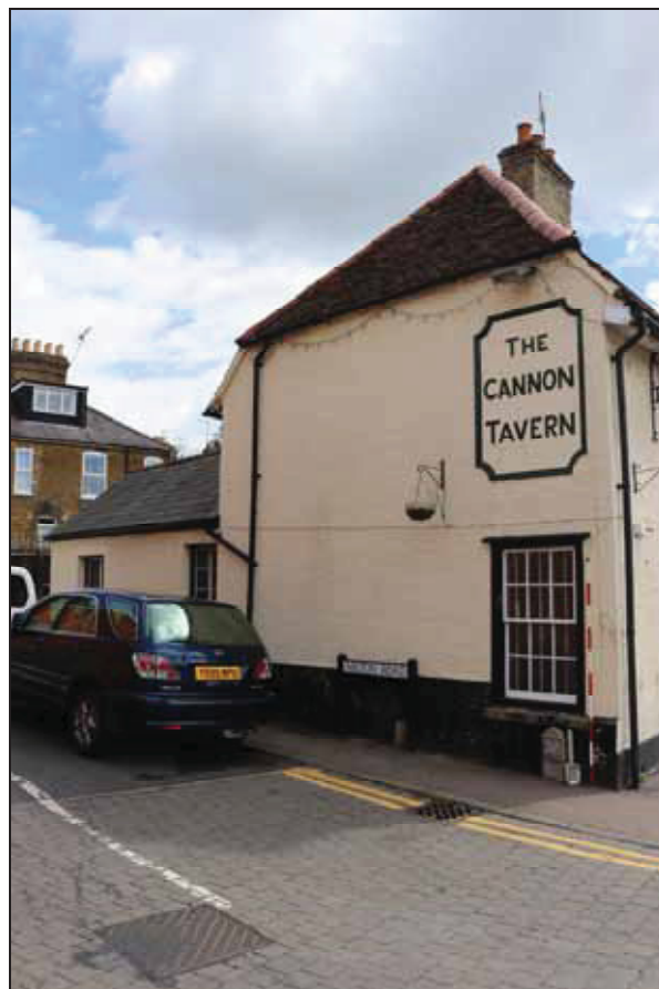
Plate 2 Exterior of Building 1, taken from the south-west (DP 10)
