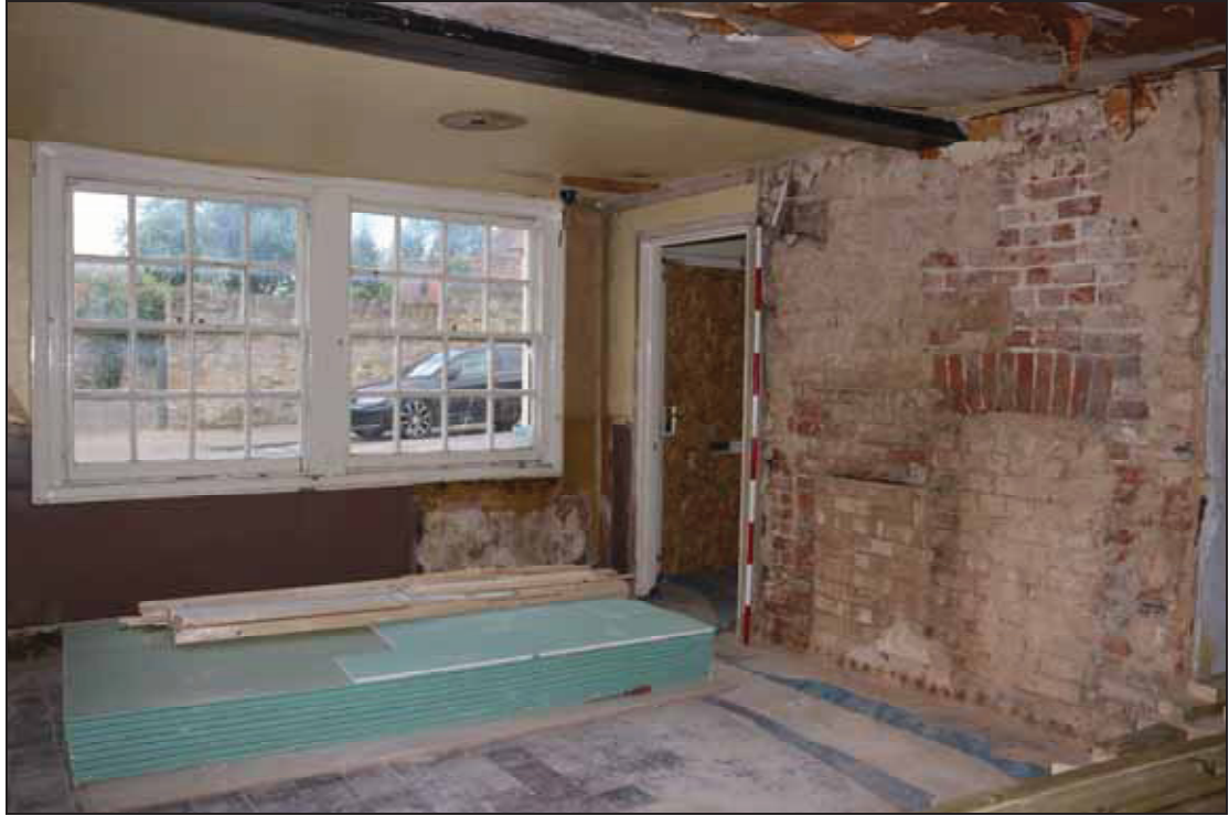
Plate 5 Interior of GF01 in Building 1, taken from the north-east (DP 26)
