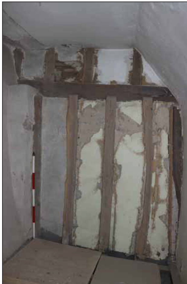
Plate 16 Timber-framing in FF01a in Building 1, taken from the west (DP 65)
