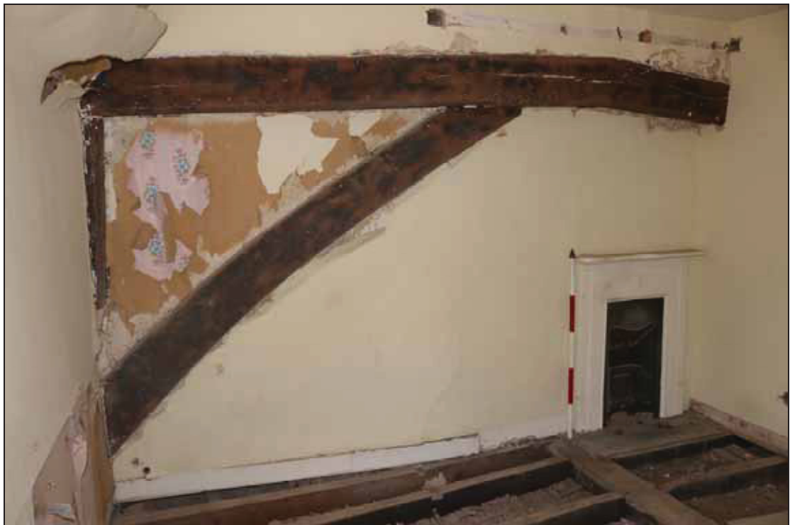
Plate 18 Interior of FF03 in Building 1, taken from the south-east (DP 74)
