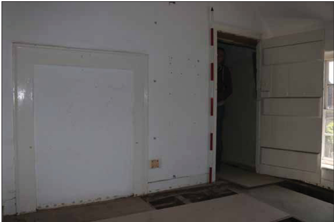
Plate 14 Interior of FF01 in Building 1, taken from the north-west (DP 62)
