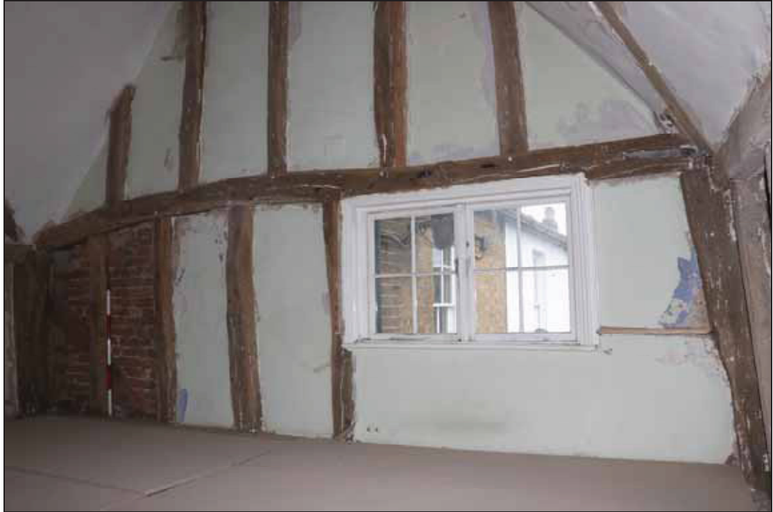
Plate 23 Timber-framing in FF04 in Building 1, taken from the south-east (DP 90)
