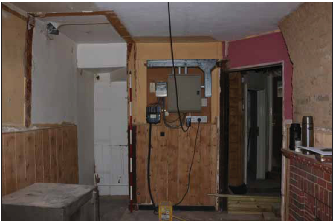
Plate 10 Interior of GF02 in Building 1, taken from the south (DP 22)
