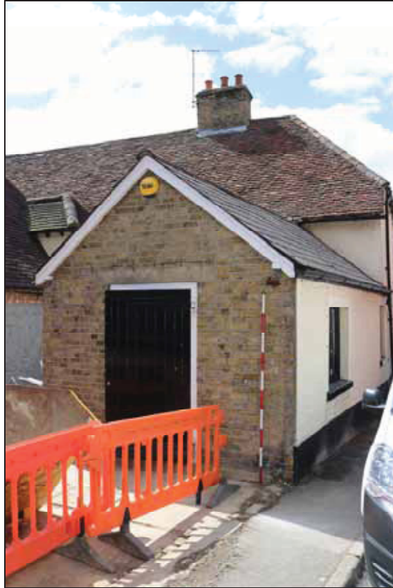
Plate 3 Rear outshot to Building 1, taken from the north (DP 12)
