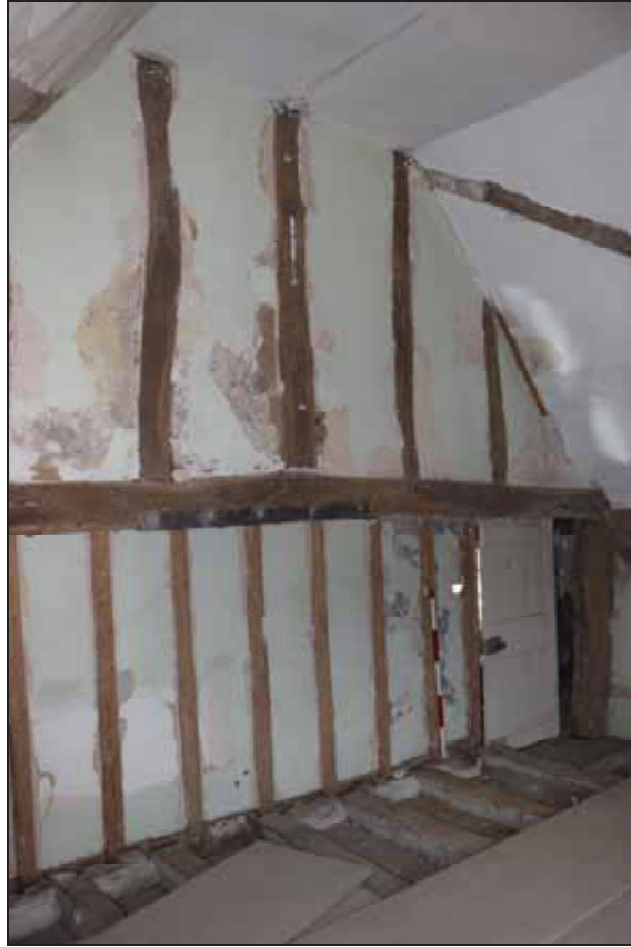
Plate 19 Timber-framing in FF04 in Building 1, taken from the south-east (DP 79)
