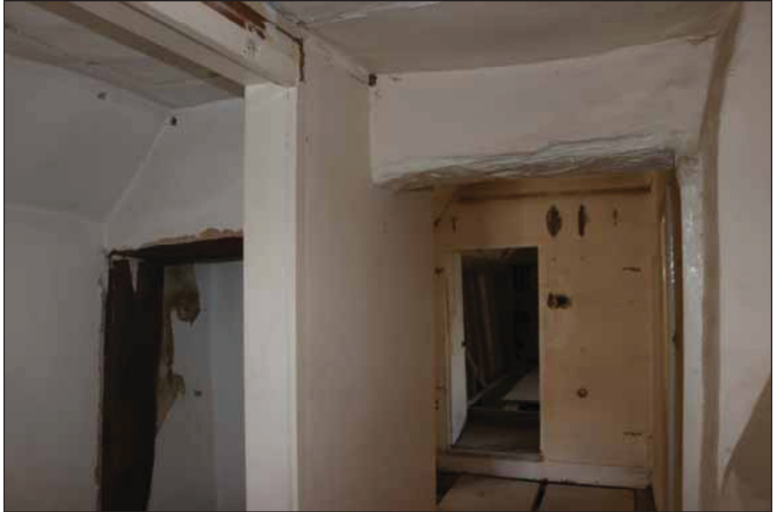
Plate 17 View of FF02 in Building 1, taken from the west (DP 103)
