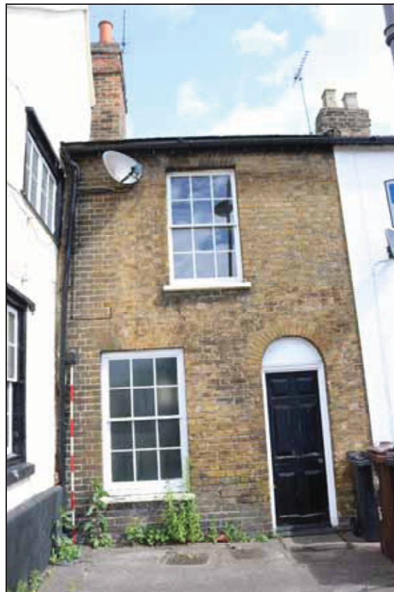
Plate 26 Exterior of Building 2, taken from the south-east (DP 03)
