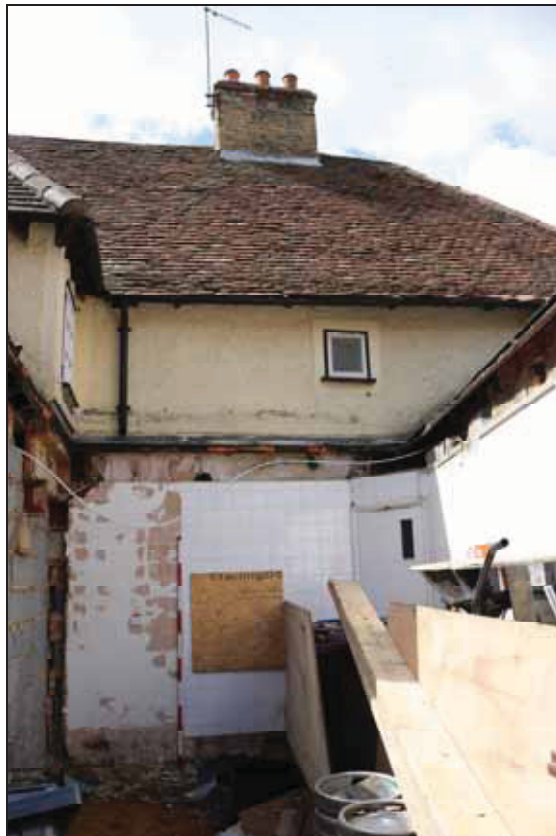
Plate 4 Rear of Building 1, taken from the north (DP 15)
