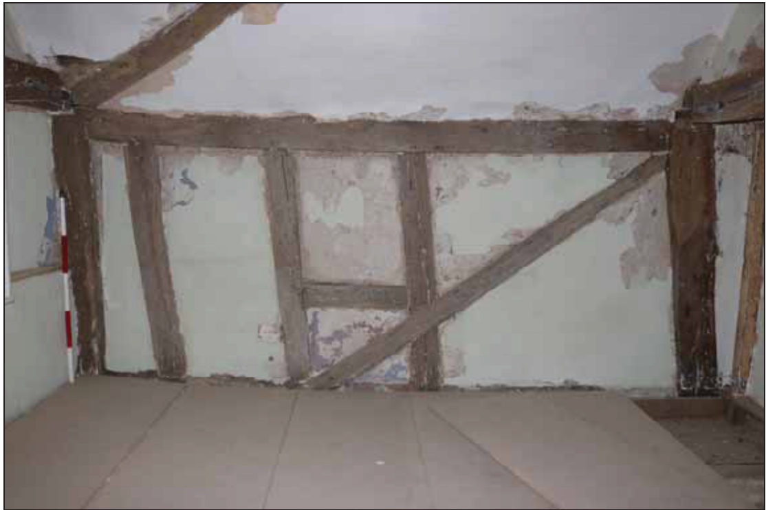
Plate 22 Timber-framing in FF04 in Building 1, taken from the south-east (DP 92)
