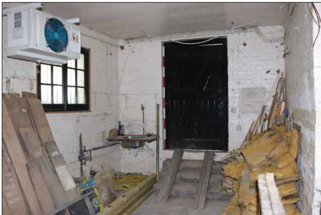
Plate 12 Interior of GF03 in Building 1, taken from the south (DP 17)
