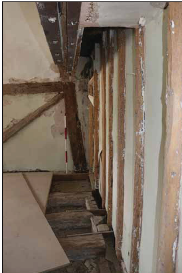
Plate 24 Timber-framing in FF04 in Building 1, taken from the south-east (DP 84)
