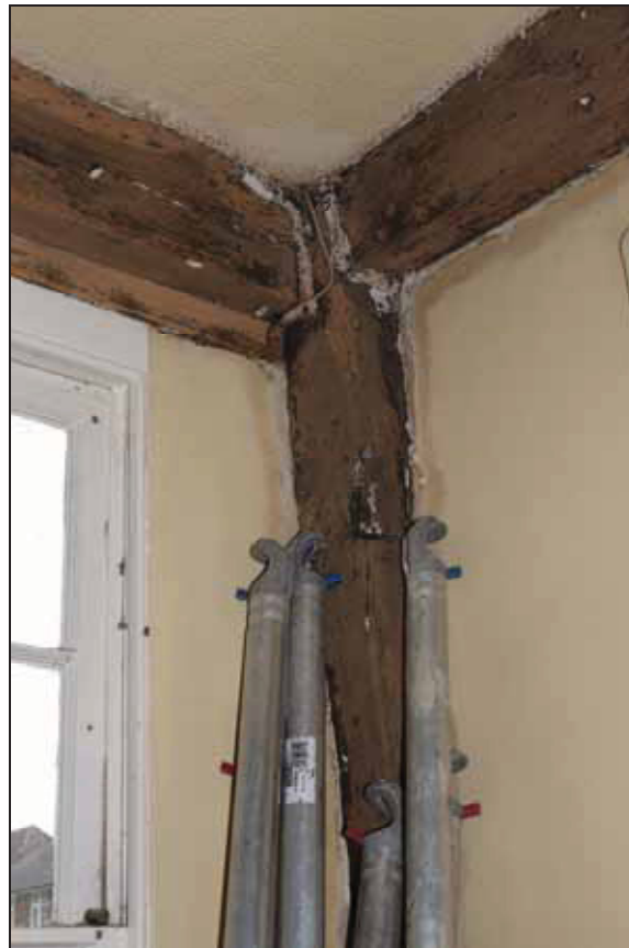
Plate 8 Timber-framing in GF01 in Building 1, taken from the north-west (DP 41)
