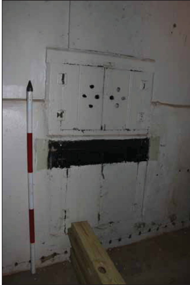
Plate 13 Small cupboard in GF03 in Building 1, taken from the north (DP 19)
