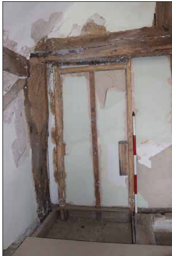
Plate 20 Former doorway in FF04 in Building 1, taken from the east (DP 85)
