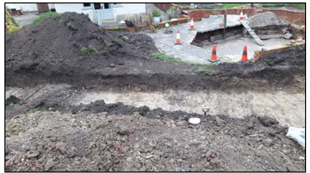
8 View of site showing a large pit
