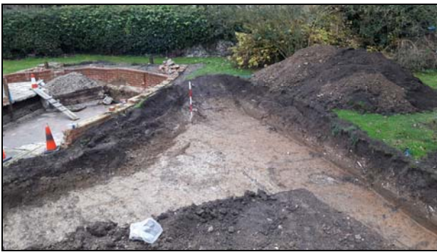
7 General view of site
