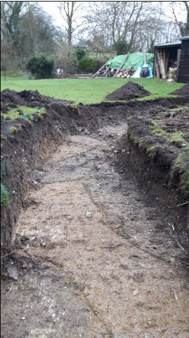
3 View of previous foundations
