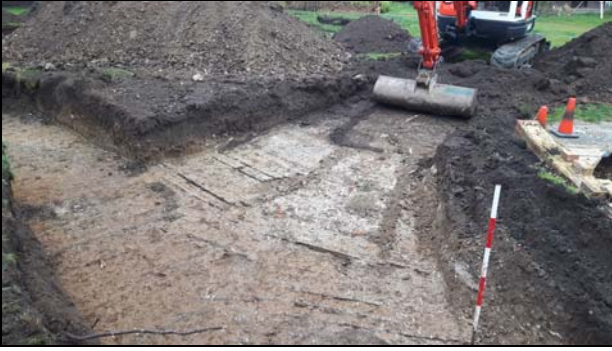
1 Trench being excavated
