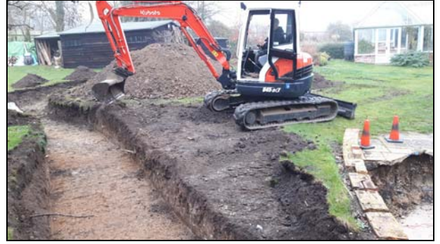
2 Trench being excavated
