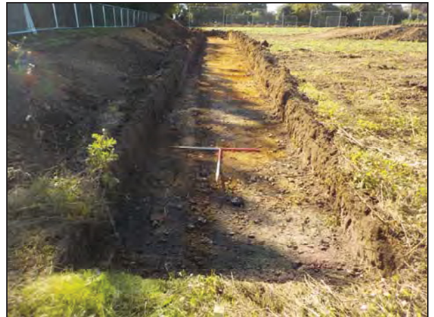
52 Trench 9 looking south-west
