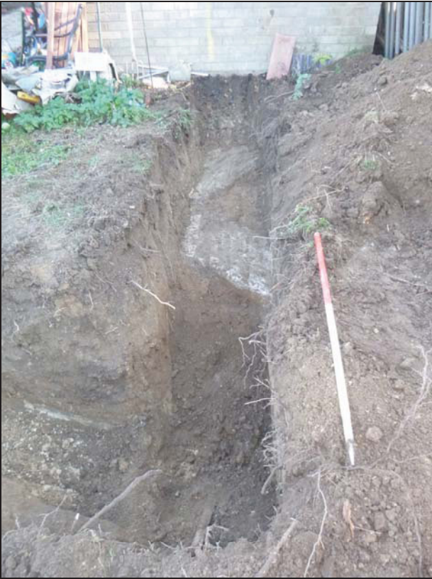
7 Concrete footings in Trench 1 looking north-east
