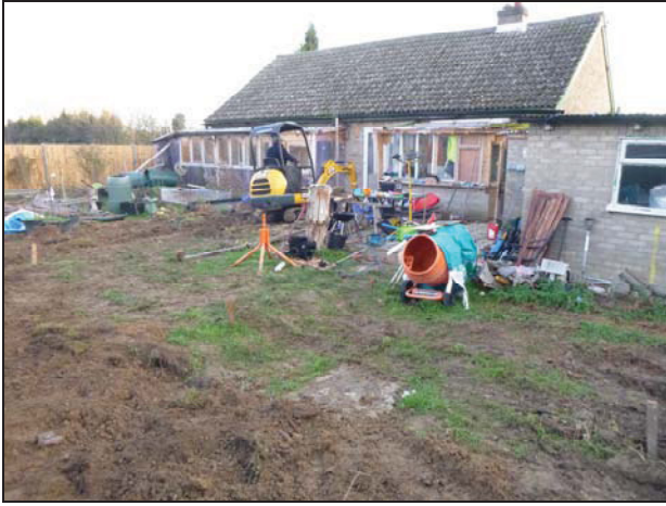
1 General site overview looking north-east
