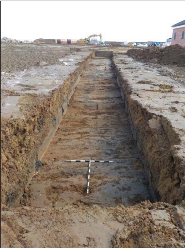
87 Trench 16 looking east
