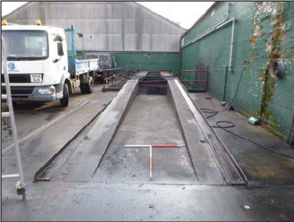
3 Chassis wash looking south-east
