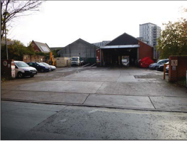
1 Main gateway looking south-east
