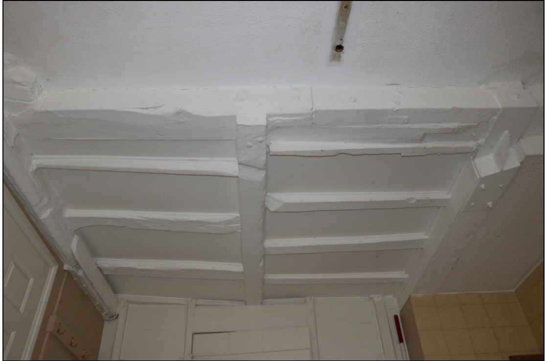
Plate 15 Detail of ceiling and face-halved scarf joint in GF03, taken from the north-west (DP 044)
