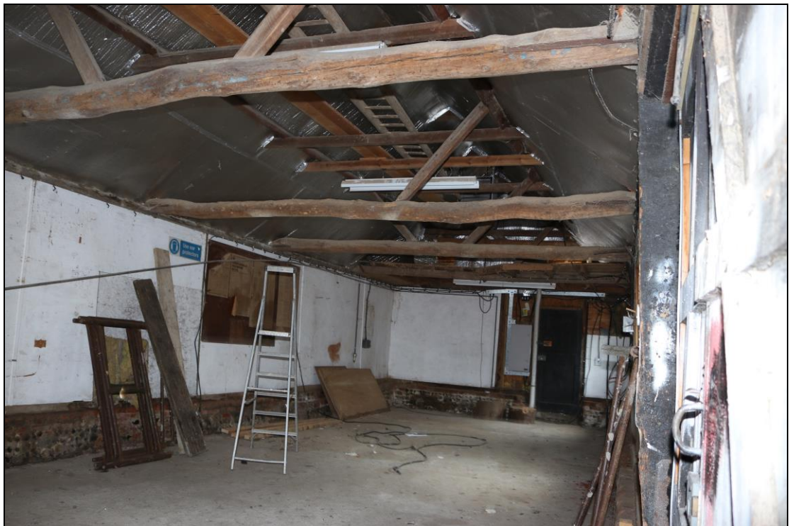
Plate 48 Interior of Outbuilding 1, Unit 1, taken from the east (DP 124)
