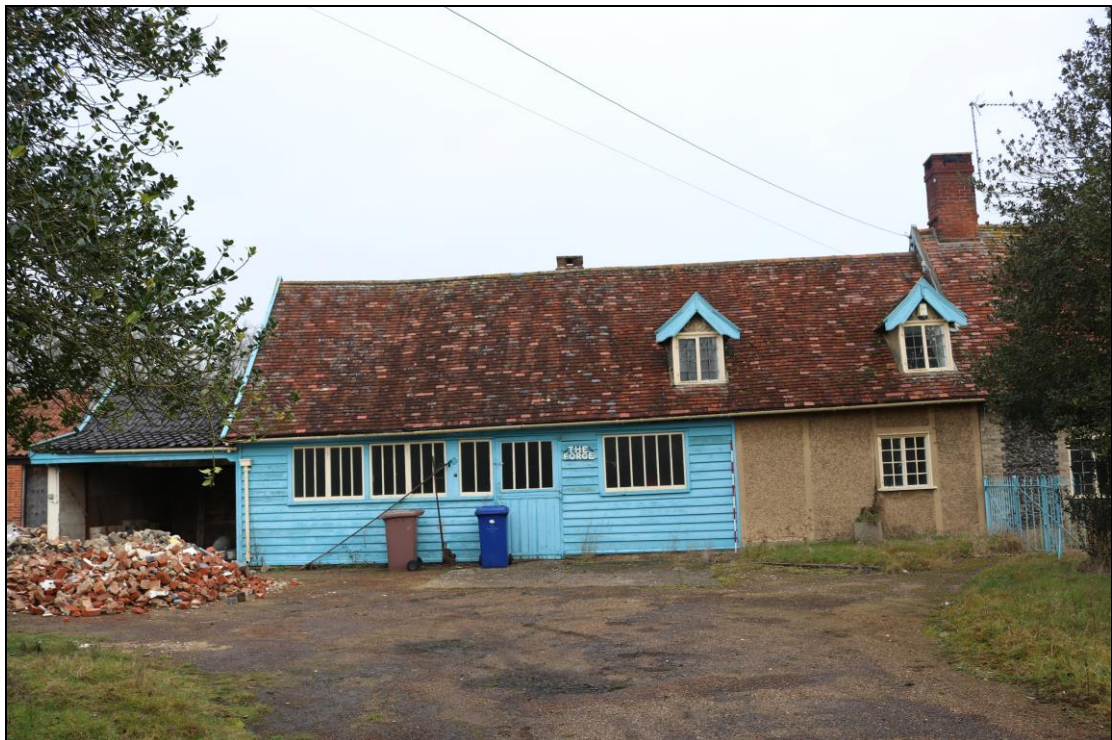
Plate 2 Exterior of the Cartshed and Workshop, taken from the south-east (DP 010)
