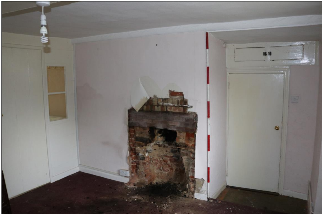
Plate 14 North-eastern wall of GF02, taken from the south-west (DP 037)
