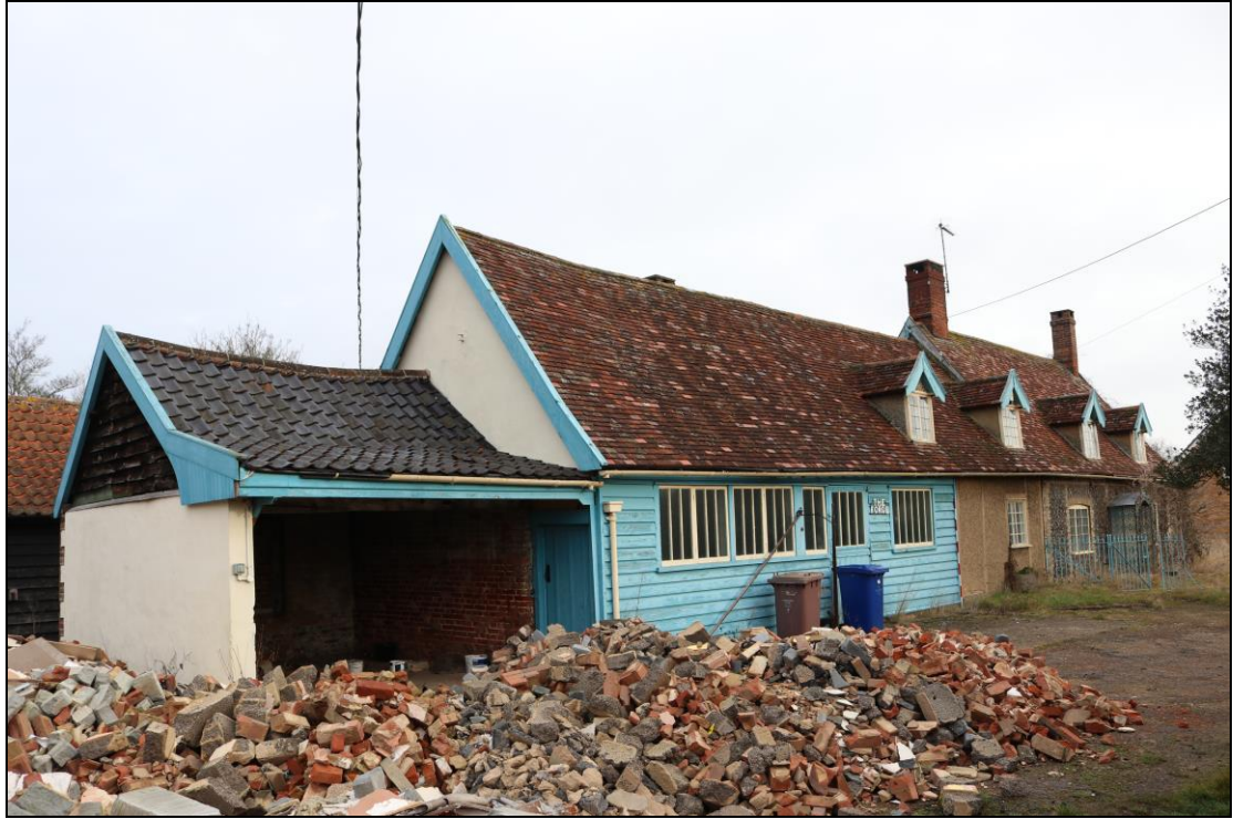
Plate 3 Exterior of the building, taken from the south-west (DP 001)
