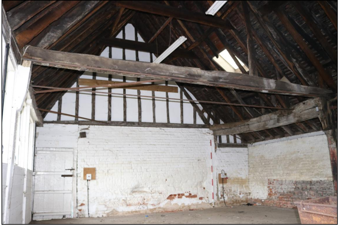
Plate 35 Interior of GF11, taken from the east (DP 120)
