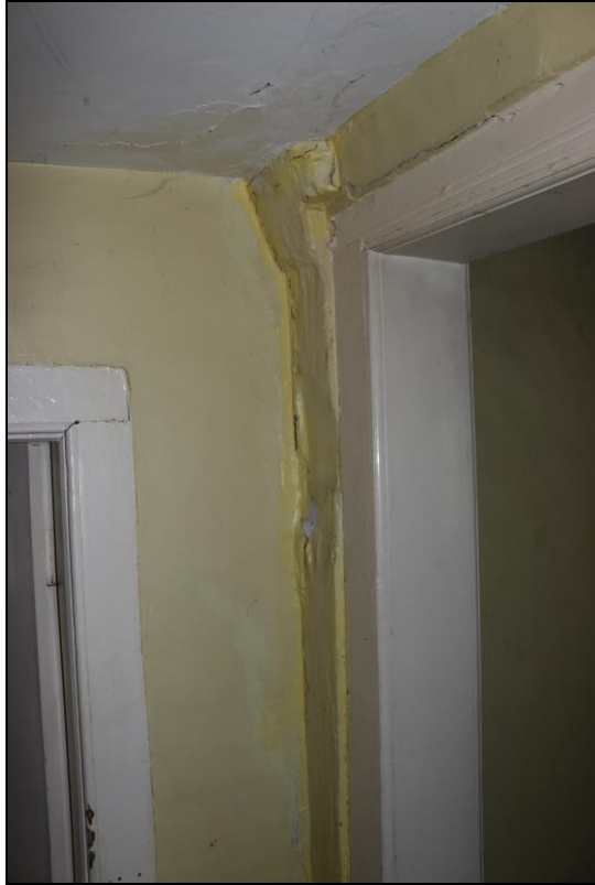
Plate 21 Detail of two splayed jowled bay posts in GF08, taken from the west, and south west (DP 052 & 056)
