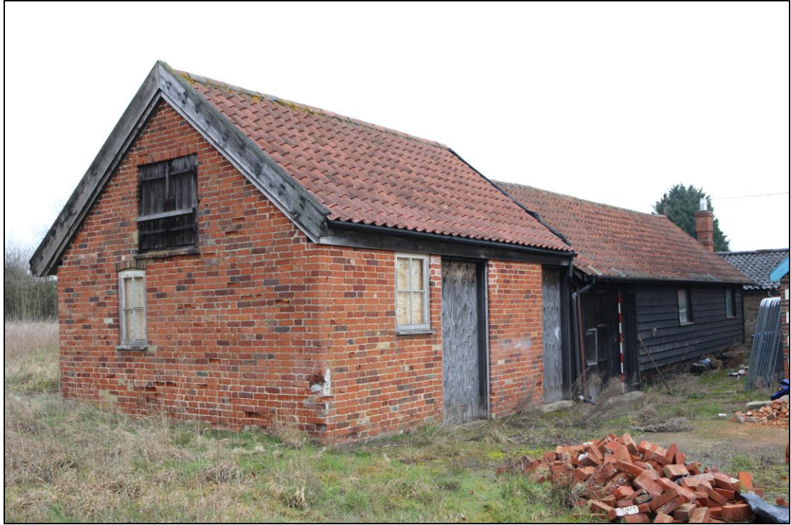
Plate 47 Exterior of Outbuilding 1, taken from the south-west (DP 018)
