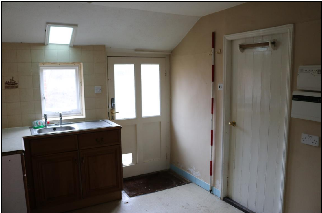
Plate 16 Interior of GF03, taken from the south (DP 045)
