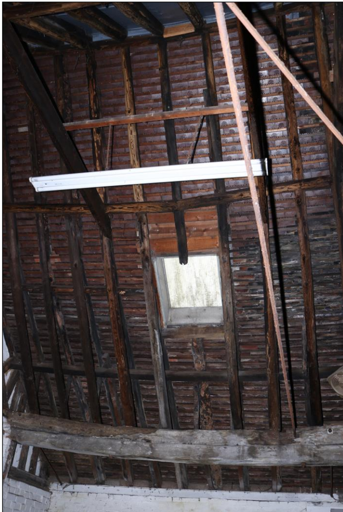
Plate 36 Northern roof pitch over GF11, taken from the south-east (DP 103)
