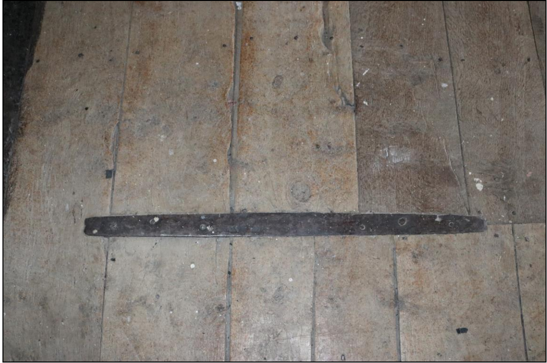
Plate 37 Detail of the floorboards in FF01, taken from the north-east (DP 068)
