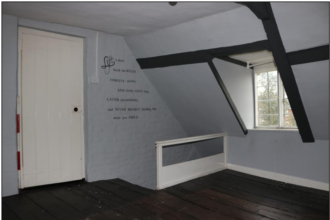
Plate 44 Interior of FF04, showing timber framed elements and the joggled butt-purlin roof form, taken from north-west (DP 064)
