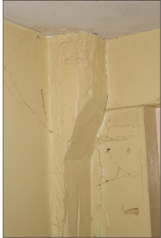
Plate 21 Detail of two splayed jowled bay posts in GF08, taken from the west, and south west (DP 052 & 056)
