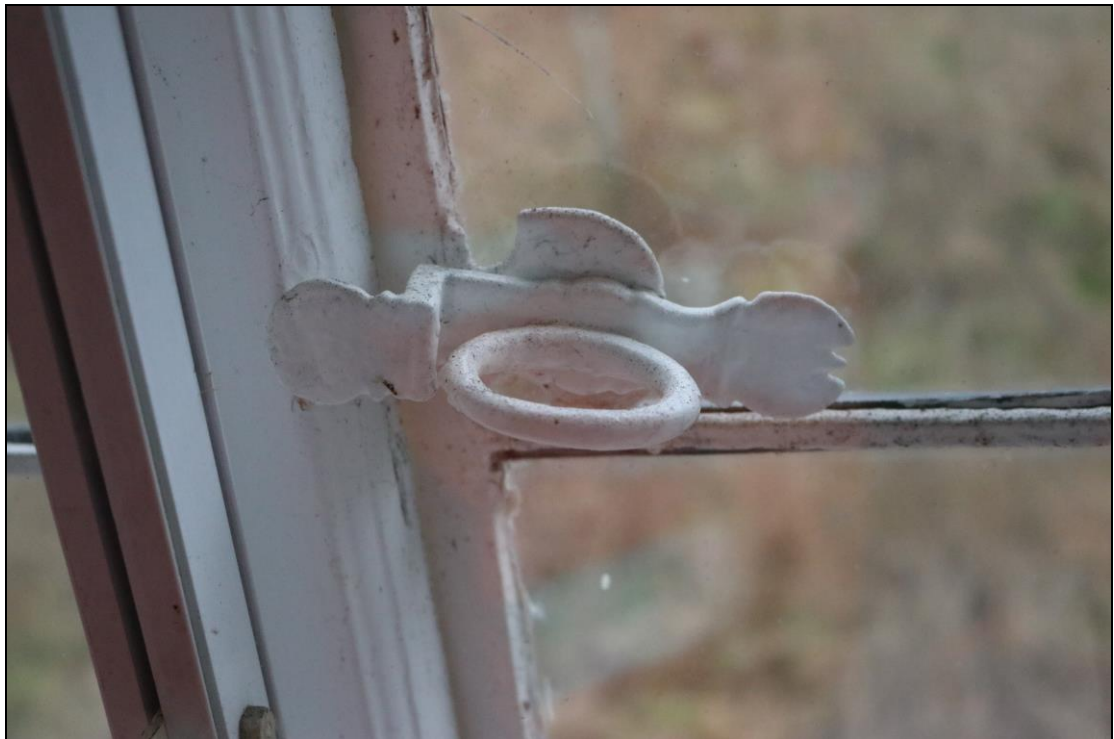
Plate 46 Detail of turnbuckle window catch in FF02, taken from the south-west (DP 081)
