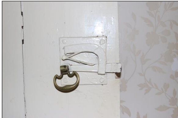
Plate 9 Boarded door to the staircase from GF01, taken from the east, and detail of a spring latch with brass drop handle on the door from GF01 to the staircase, taken from the south-east (DP 031 & 029)
