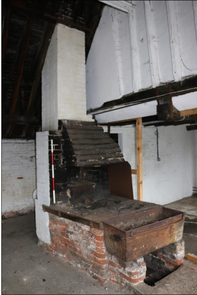
Plate 31 View of the forge in GF10, taken from the south (DP 092)
