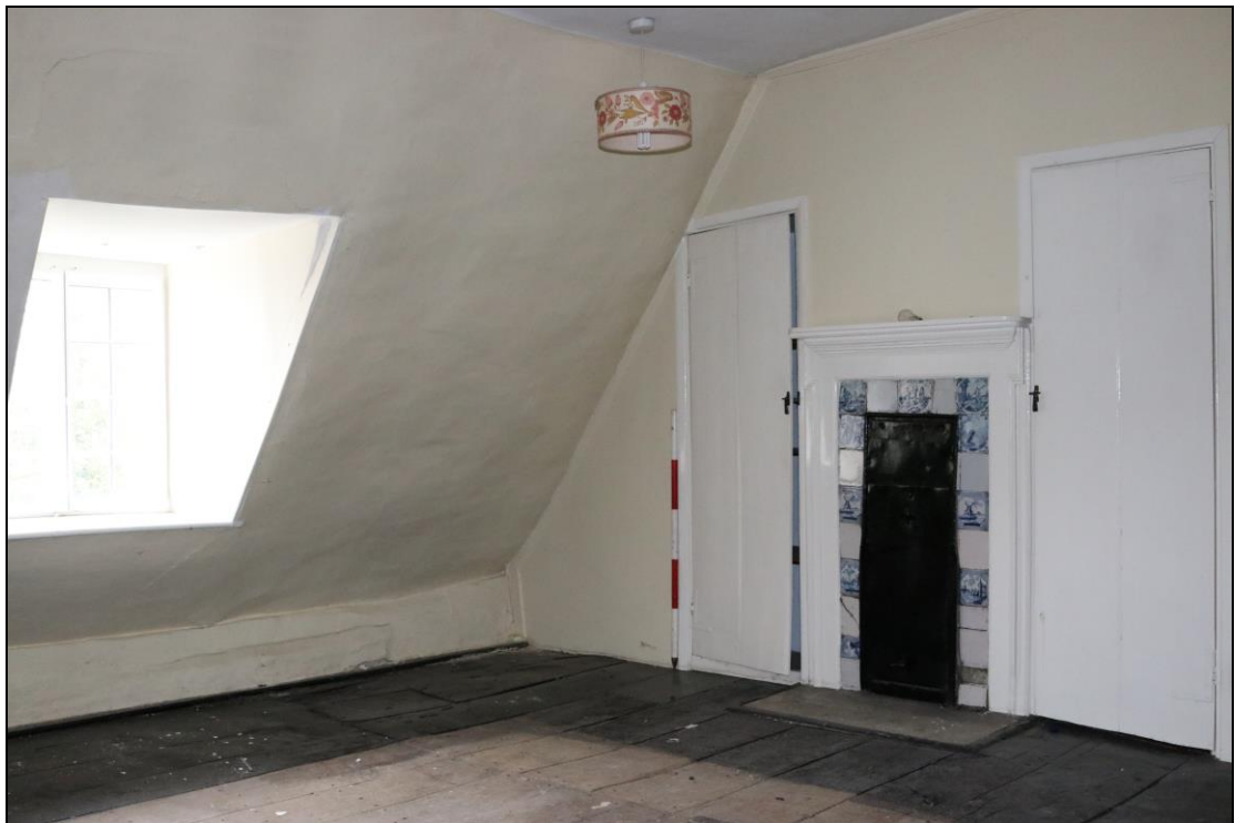
Plate 38 Interior of FF01, taken from the north (DP 067)
