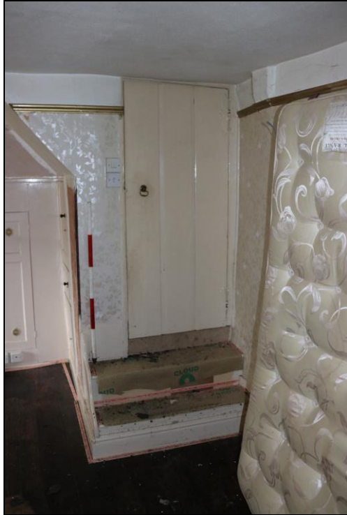
Plate 9 Boarded door to the staircase from GF01, taken from the east, and detail of a spring latch with brass drop handle on the door from GF01 to the staircase, taken from the south-east (DP 031 & 029)
