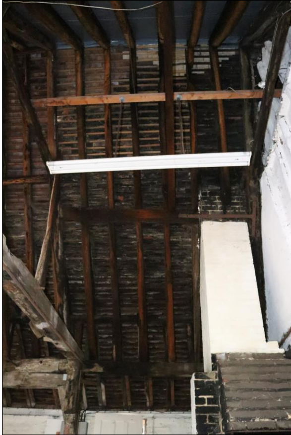
Plate 33 Northern roof pitch over GF10, taken from the south-east (DP 111)
