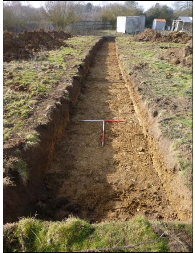
18 Trench 7 looking west
