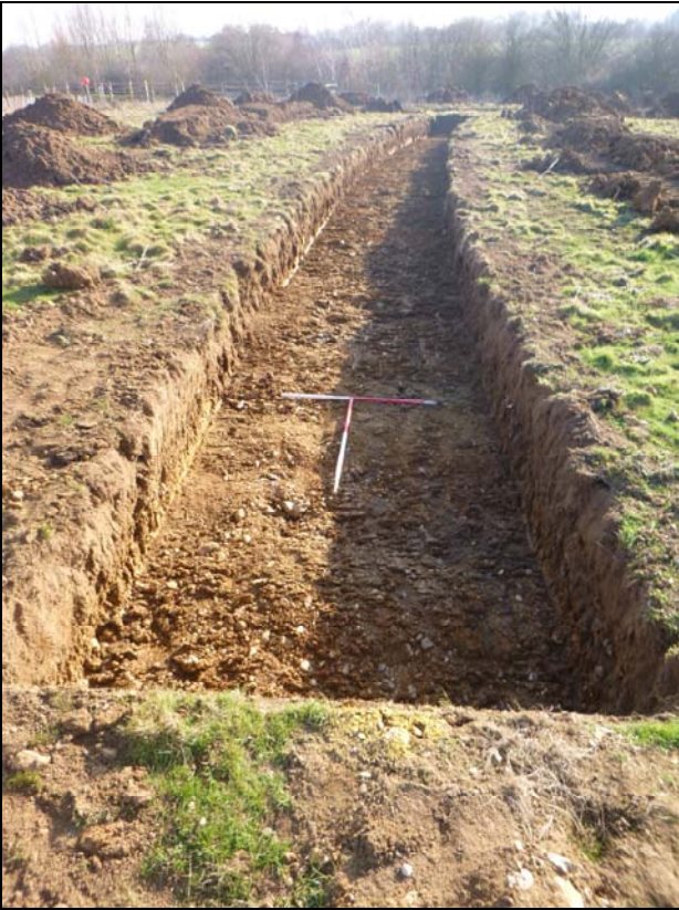
21 Trench 8 looking south
