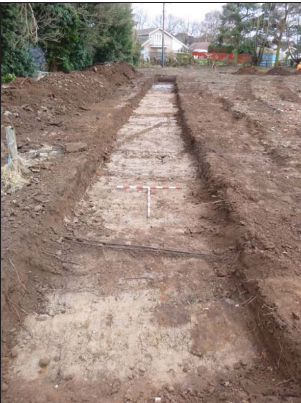
3 Trench 2 looking north-east (1m scale)
