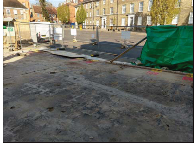
2 View of the site before commencement of works looking north-west
