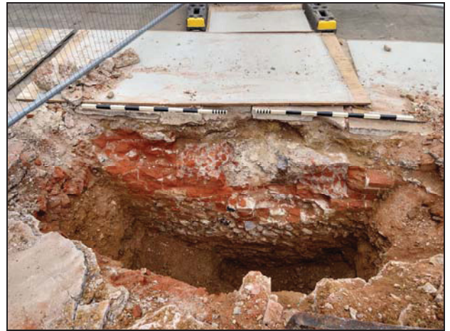
8 Test Pits 5 & 6 looking north-west showing foundations of former brick shop frontage, M2002 and flint cobble wall M2017
