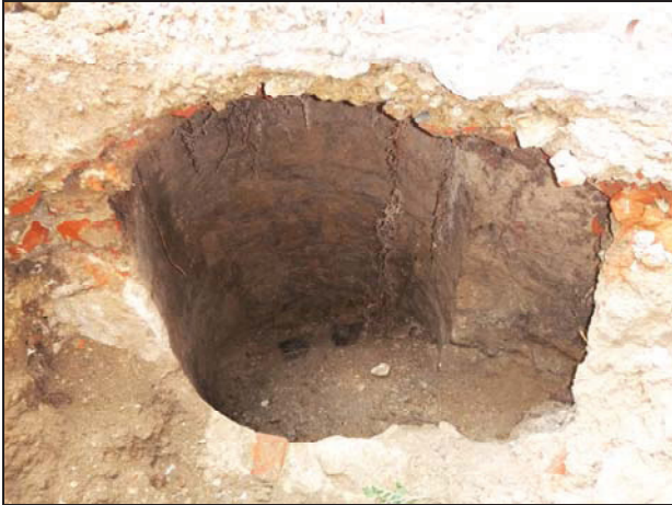
27 Test Pit 31 showing interior of soakaway M2033, with drainage channel, M2035, on the right
