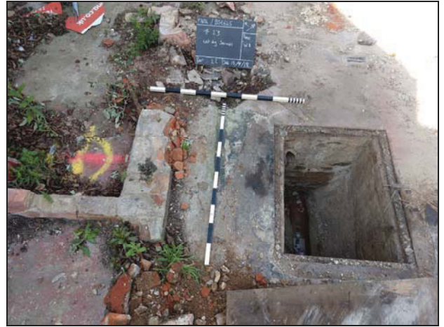
22 Test Pit 23 not dug due to services
