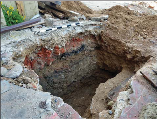
11 Test Pits 8 & 9 looking east
