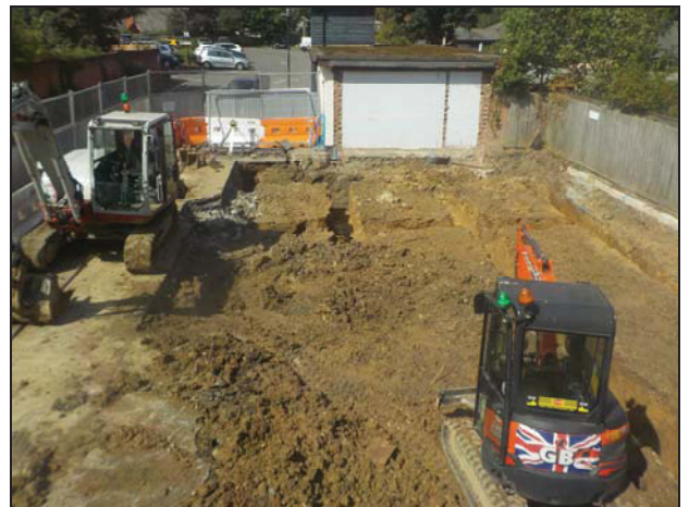
10 View of footings looking west
