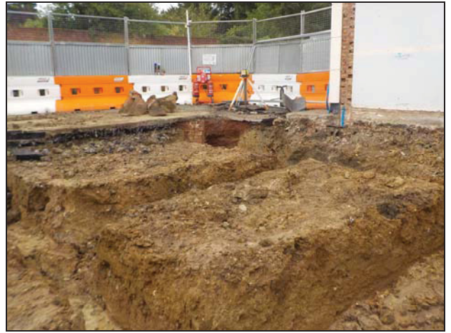
4 View of footings looking south-west
