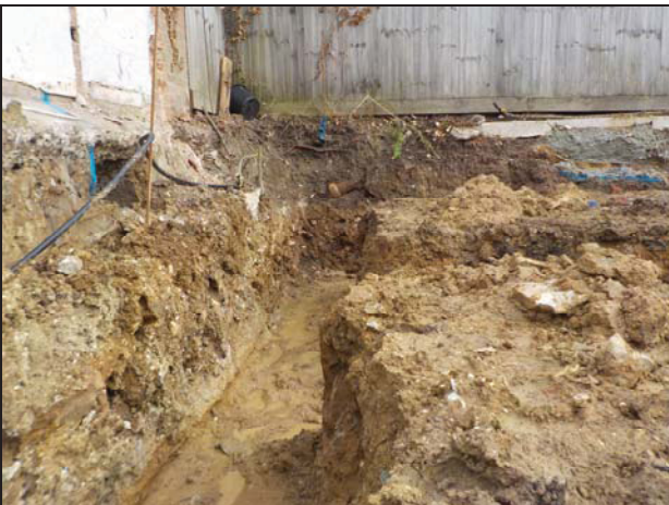
5 Detailed view of footings
