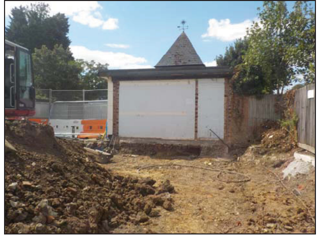
2 View of site looking west after ground reduction
