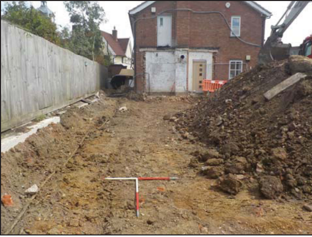
1 View of site looking east after ground reduction
