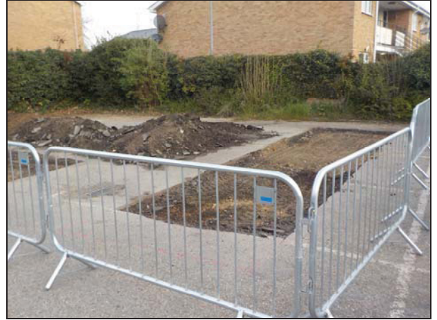
2 General site overview looking north-west
