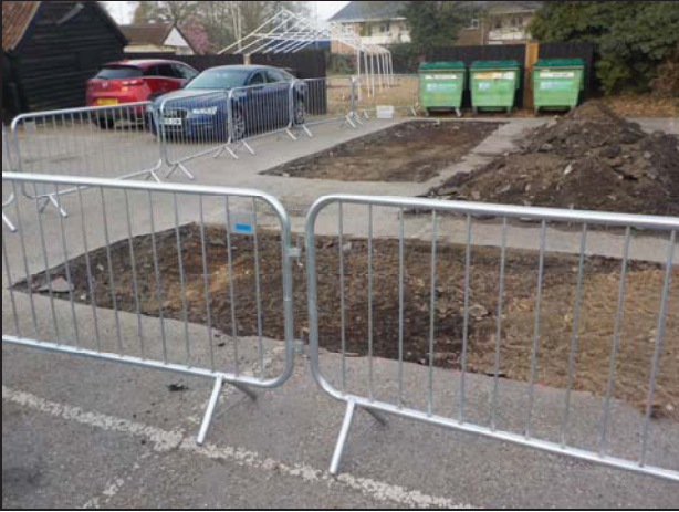
1 General site overview looking west
