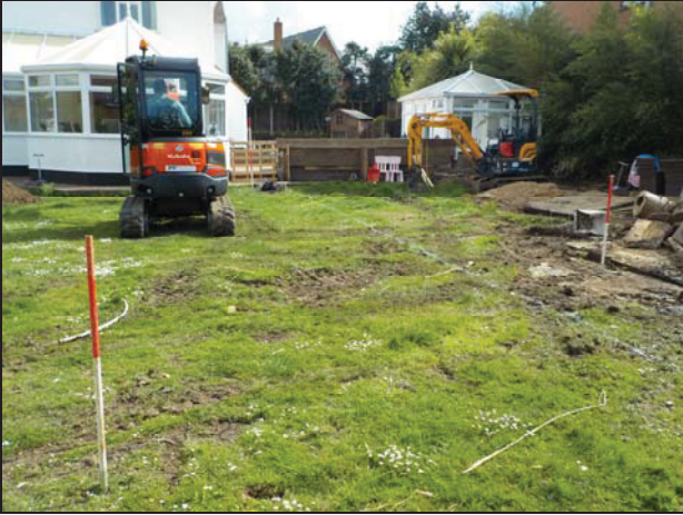
1 General site overview looking north-east
