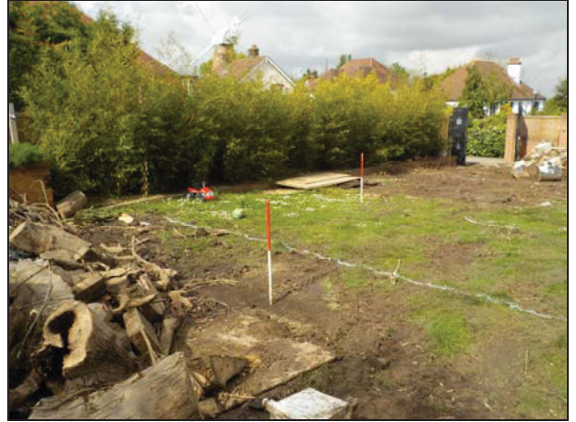
2 General site overview looking south-west
