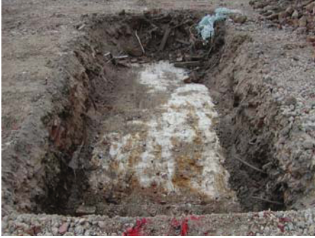
21. Trench 4b showing building rubble over natural looking south
