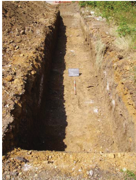
16. Trench 2 B, view west
