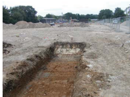
20. Trench 5 showing foundation 3009 looking west
