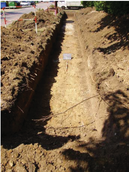
15. Trench 2 A, view west
