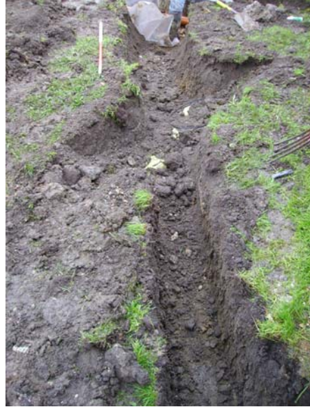
DP 8. Trench observed in watching brief, view W
