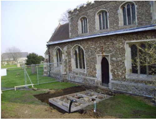
DP 1. General shot of excavation area and northern aisle, view SE
