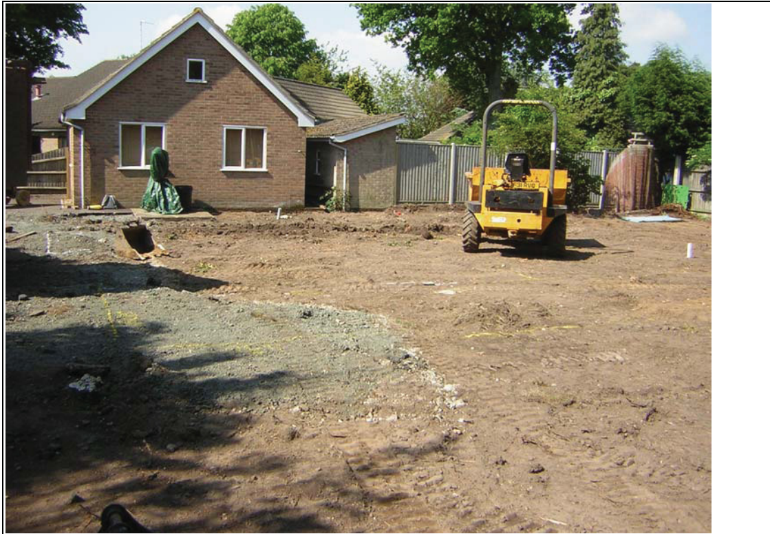
Plate 1 Site, view west (DP 1)
