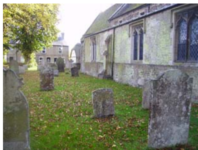
DP1 The site looking east
