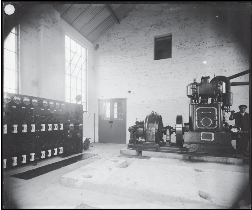
5 Room 6, Building 2. This photograph shows an electricity generator (ref. BRO_K505_1816)
