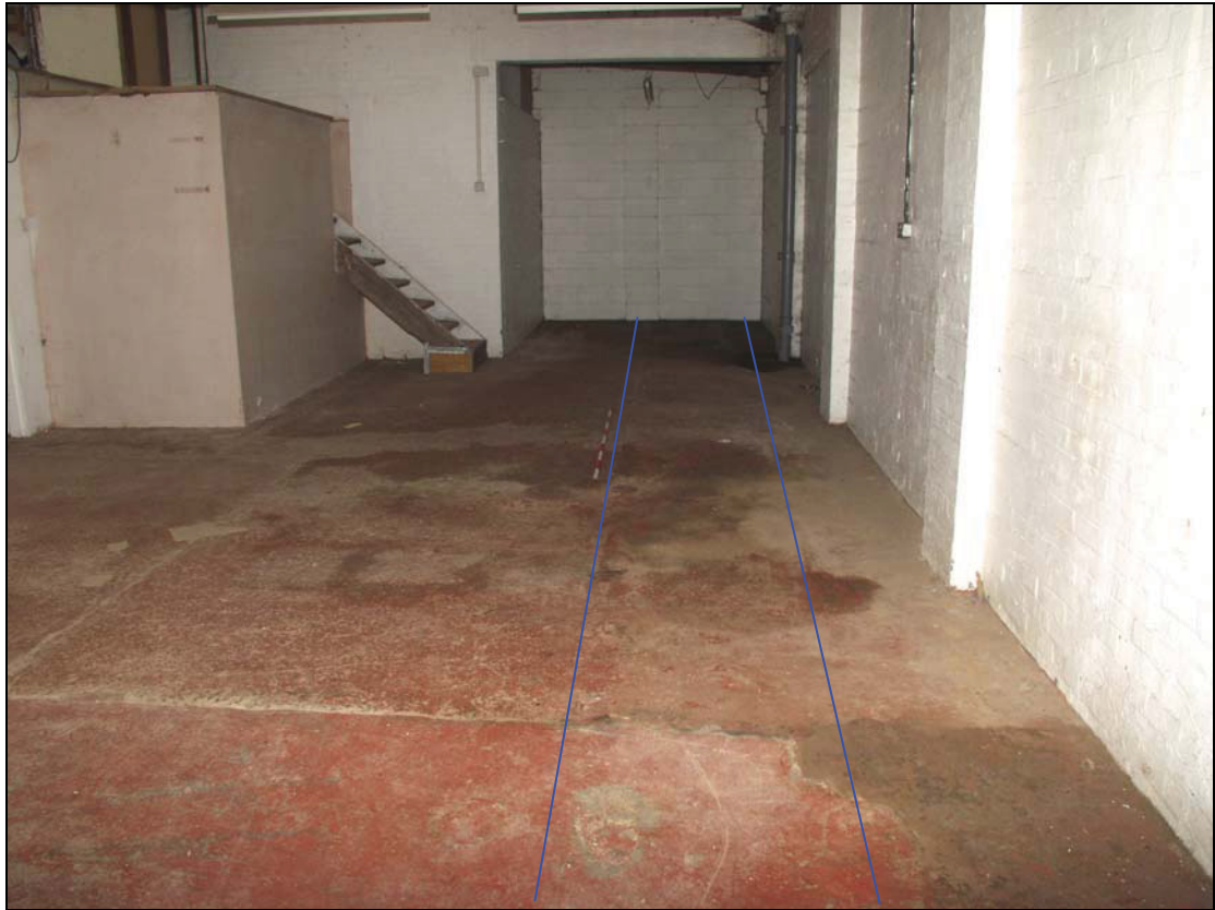
Plate 9 Line of railway tracks (highlighted) visible in floor of Unit 3, Building Group 3, taken from the west (DP 51)
