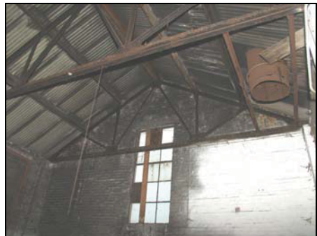
Room 2, Building 2 showing remnant of chimney flue from coal fired boiler, taken from the south-west
