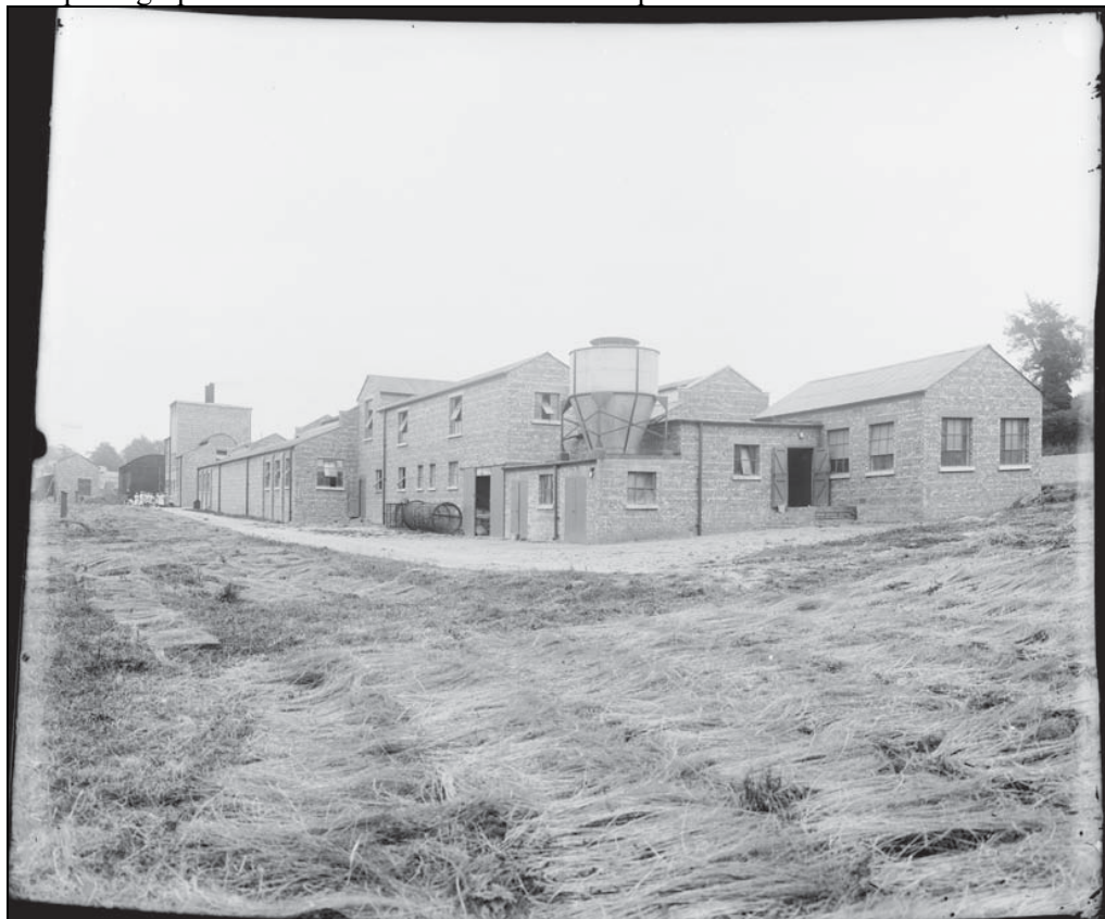
1 Building Group 3, taken from the north-west (ref. BRO_K505_1812)
