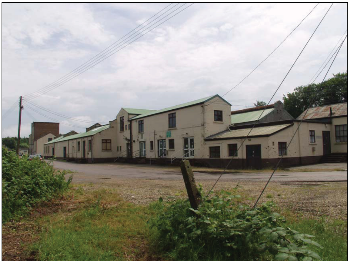
Plate 6 North and west elevations of Building Group 3, taken from the north-west (DP 24)
