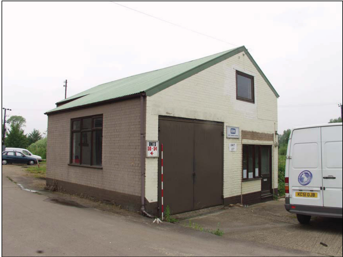
Plate 13 South and east elevations of Building 4, taken from the south-east (DP 94)
