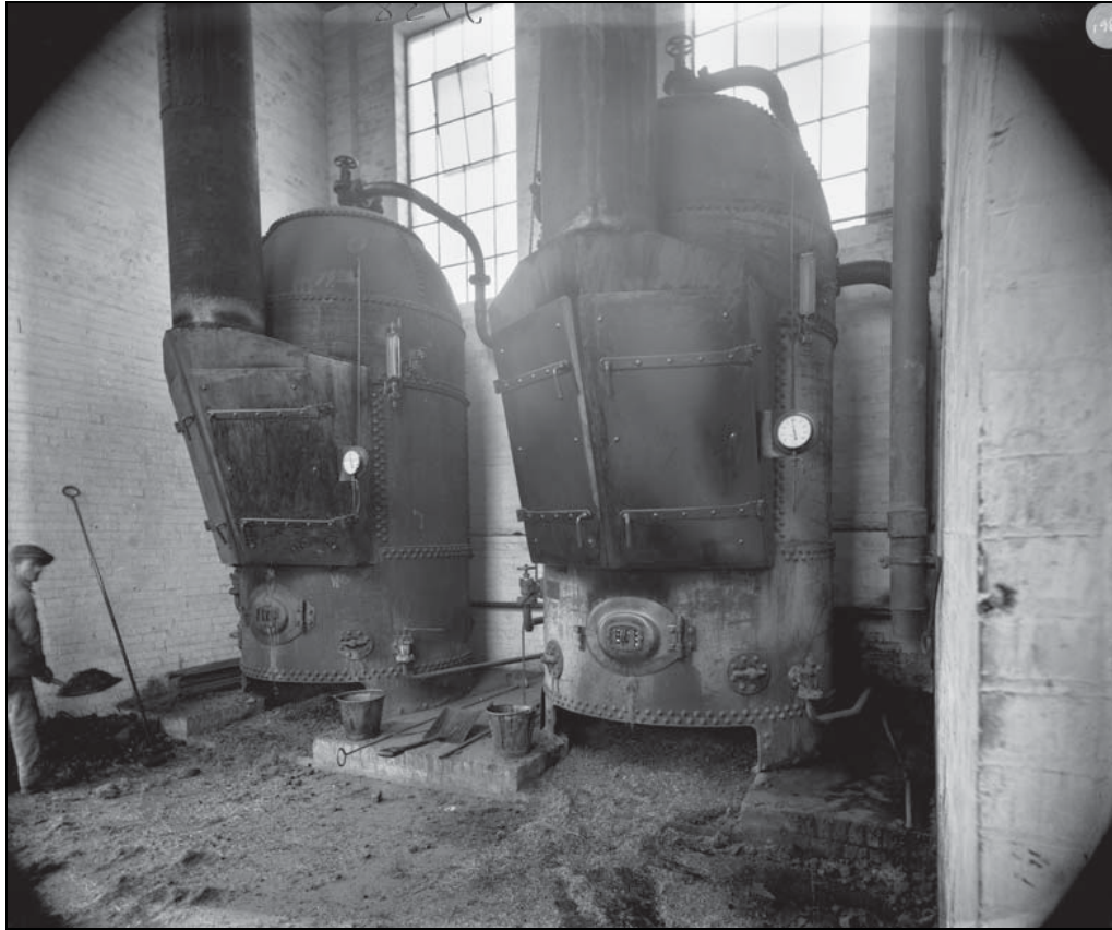
11 Coal fired boilers in Room 1, Building 2, taken from the north-west (ref. BRO_K505_1989)
