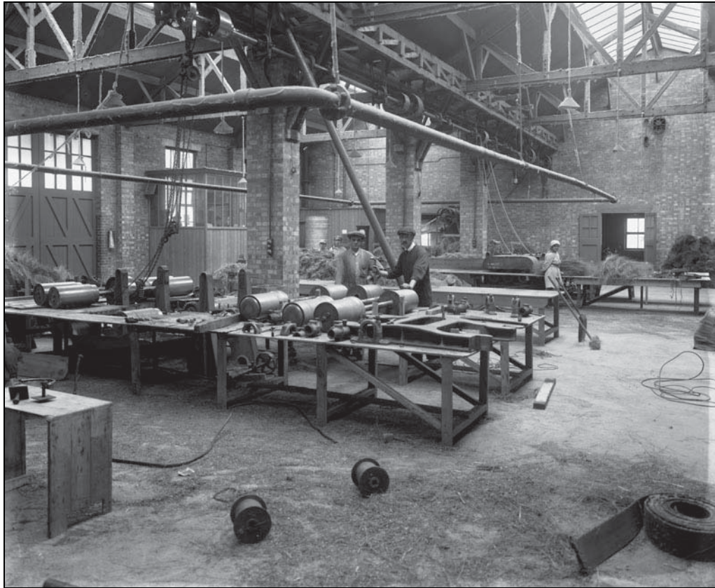
3 Unit 2, Building Group 1, taken from the south-west (ref. BRO_K505_1814)
