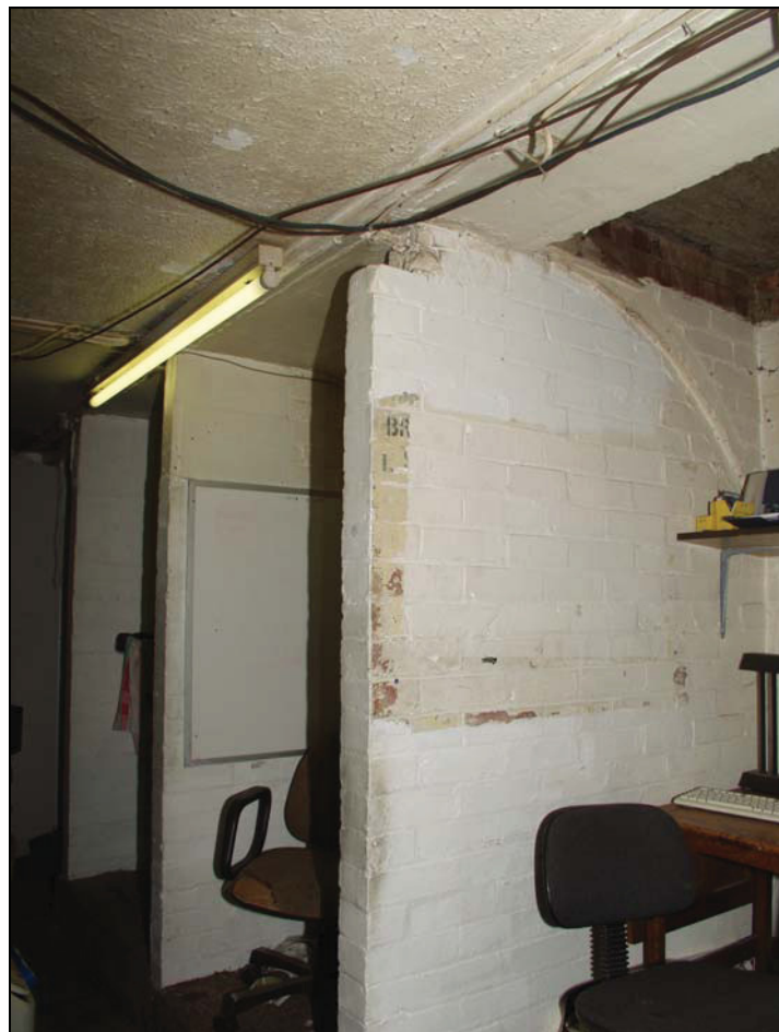
Plate 8 Unit 2, Building Group 3, taken from the north-west (DP 48)
