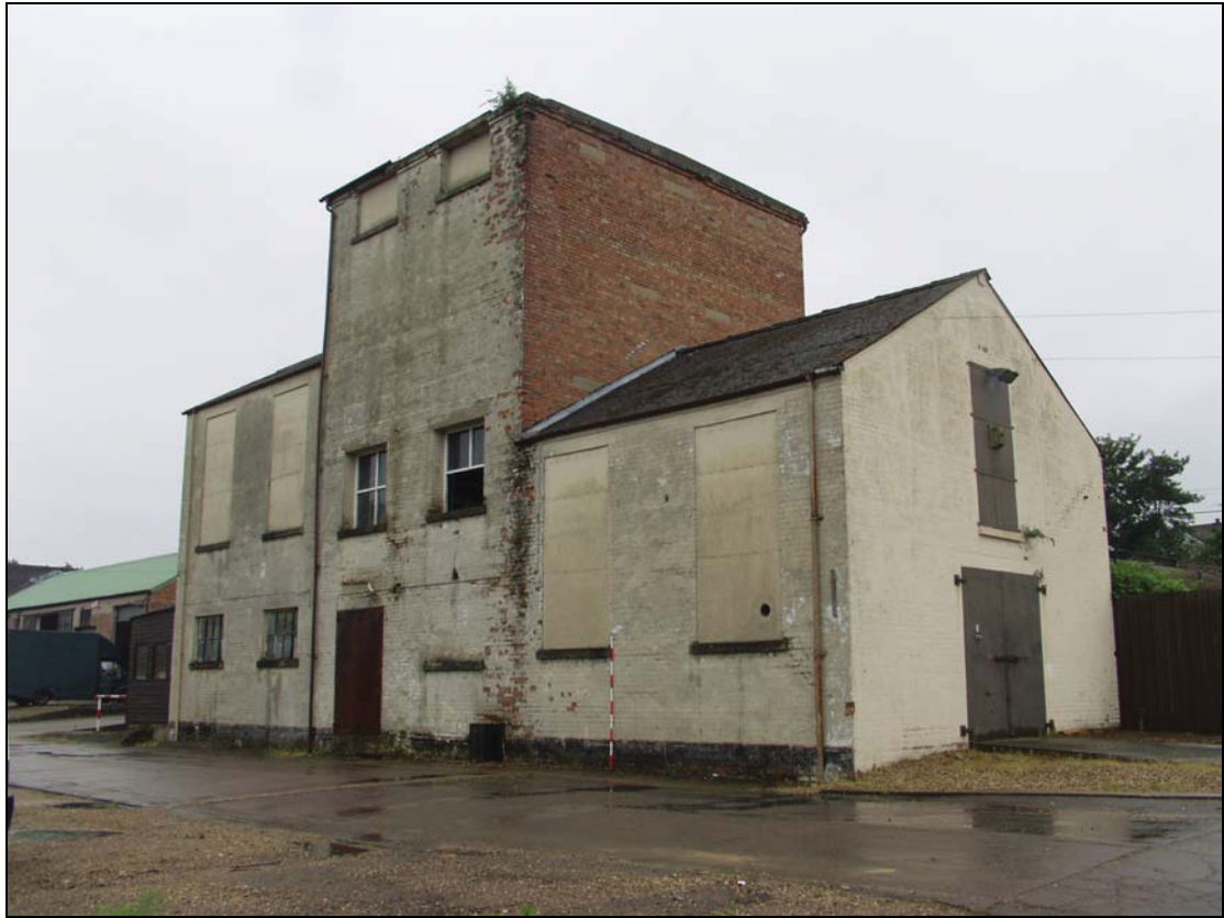
Plate 3 North elevation of Building 2, taken from the north-west (DP 19)
