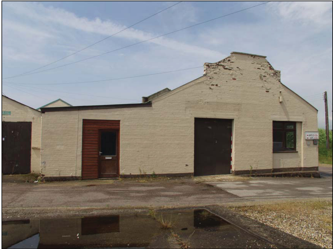
Plate 7 East elevation of Building Group 3, taken from the east (DP 30)
