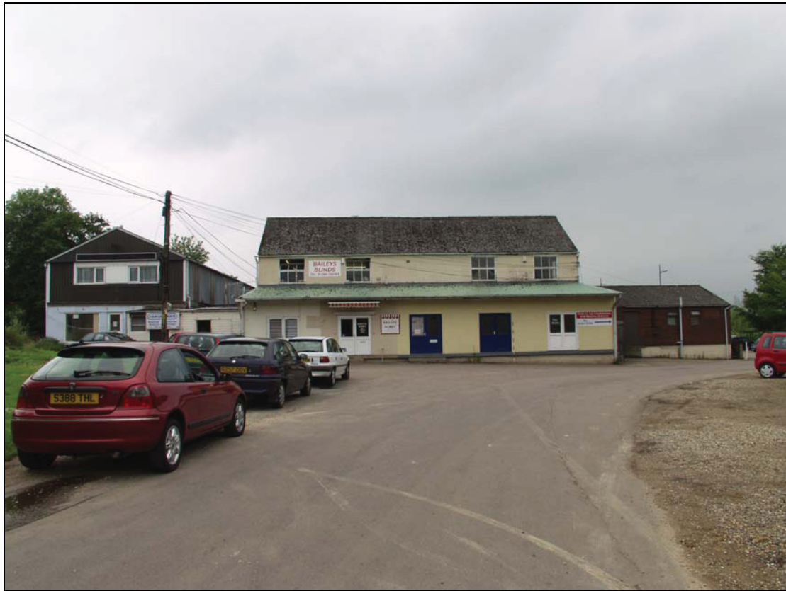
Plate 1 East elevation of Building Group 1, taken from the east (DP 77)
