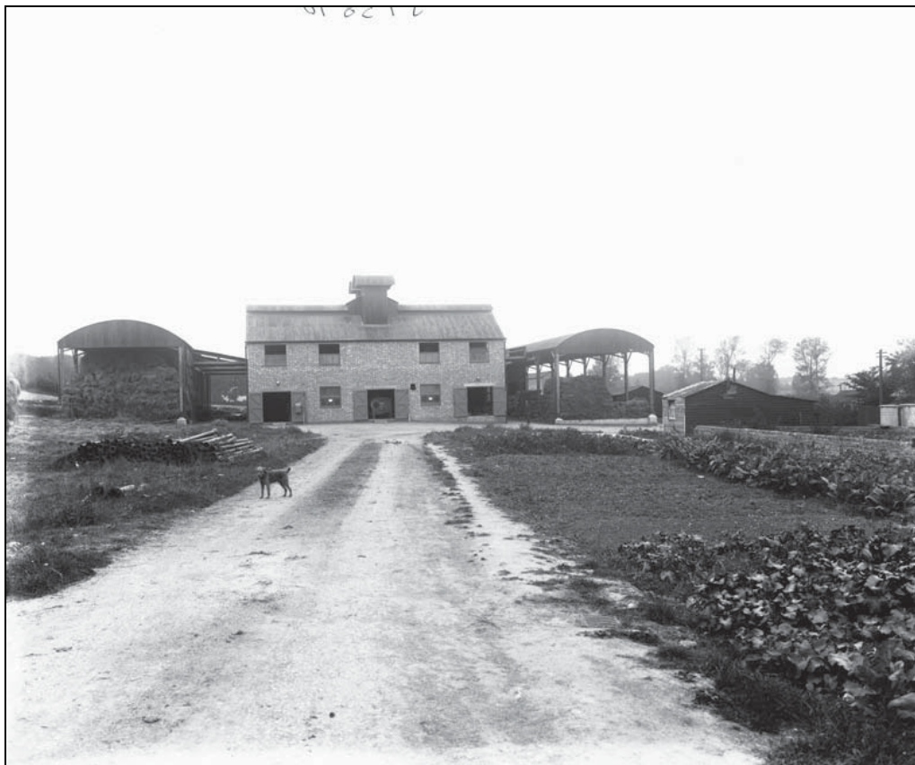
10 Building Group 1, showing flanking Dutch barns, taken from the east (ref. BRO_K505_1988)
