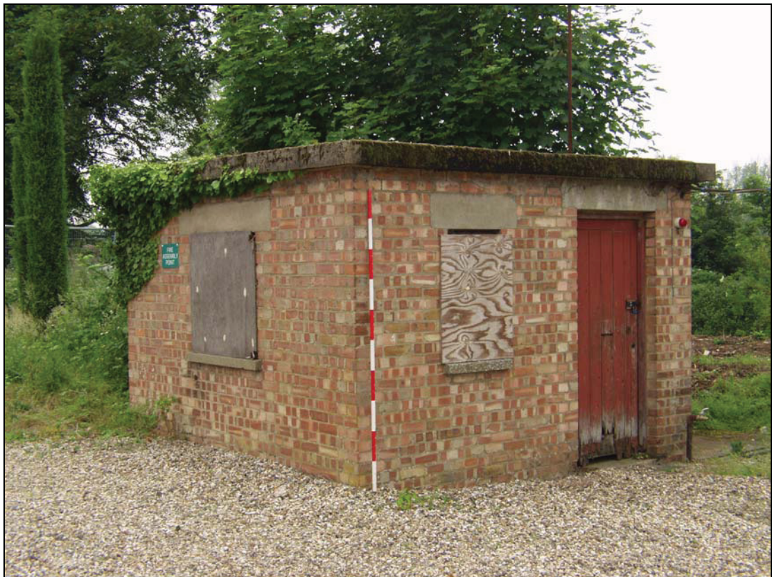
Plate 14 South and east elevations of Building 5, taken from the south-east (DP 95)
