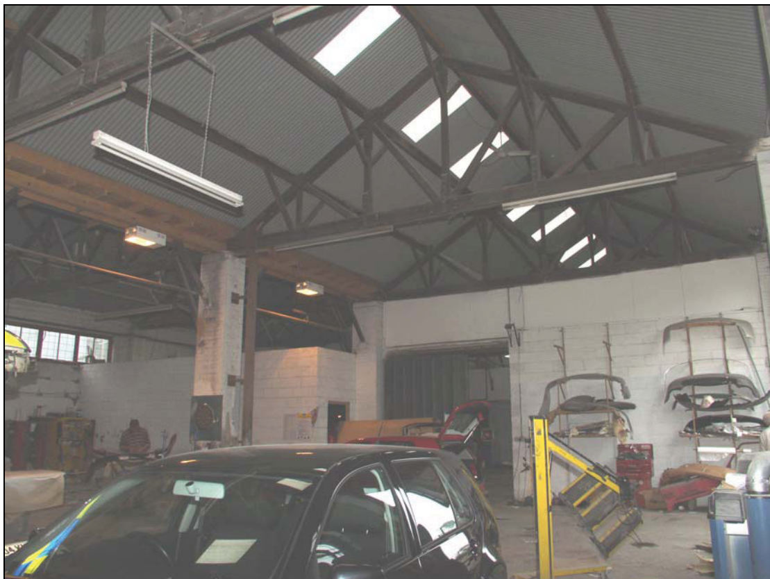
Plate 2 Unit 2, Building Group 1, taken from the north-east (DP 85)
