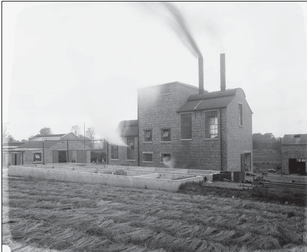
4 Building 2 and retting tanks, taken from the south-east. This photograph also shows flax laid out in the fields, part of Building Group 3 (left) and part of Building 4 (right) (ref. BRO_K505_1815)
