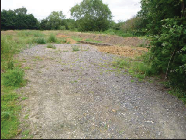
1 General site overview
