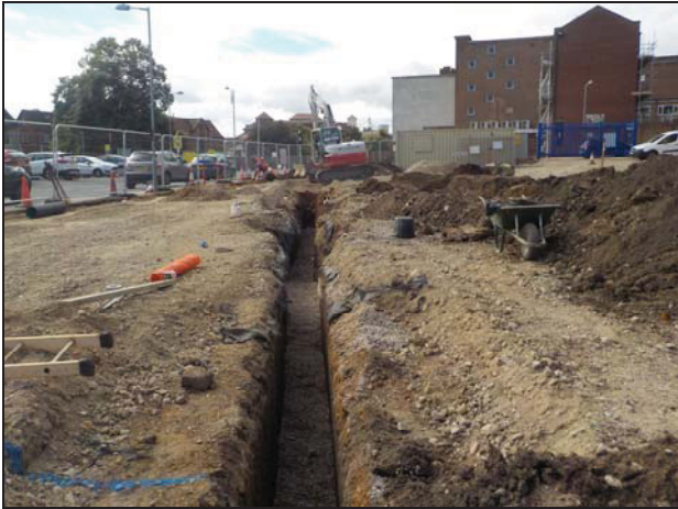
3 Main trench looking east
