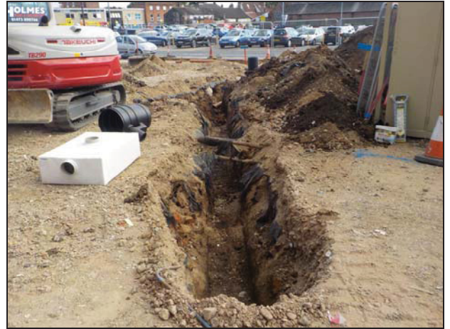
4 Western feeder drain trench looking south-east
