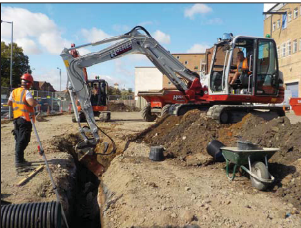
11 Breaking down concrete pillar base
