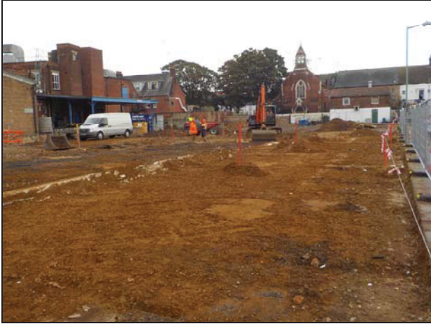
1 General site overview looking east
