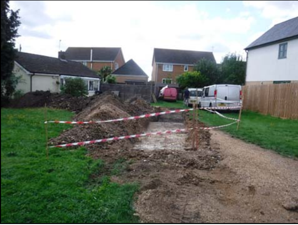
1 General site overview
