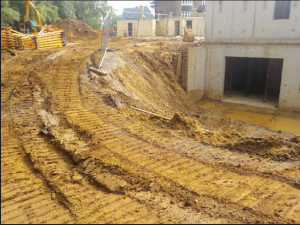
1 Area of proposed basement for Plot 2 looking north-east
